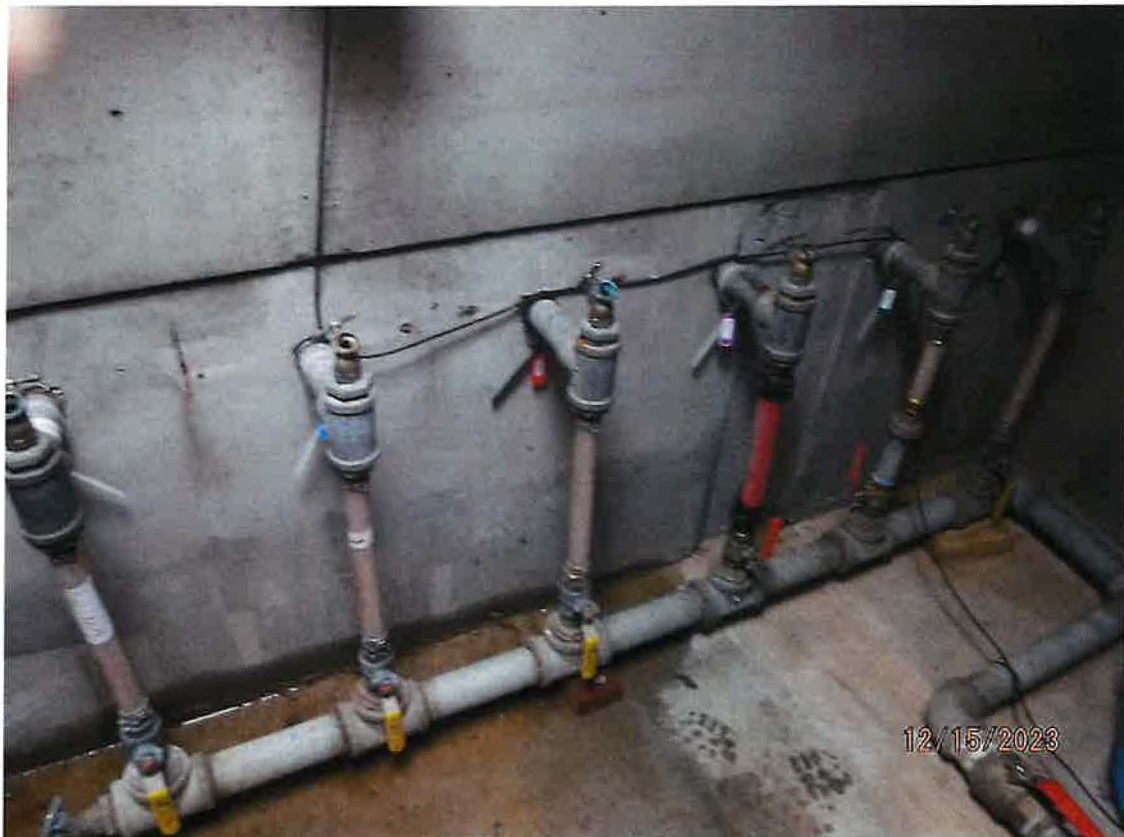
WATER LINES TO 6 HOMES WITH SHUTOFF VALVES
