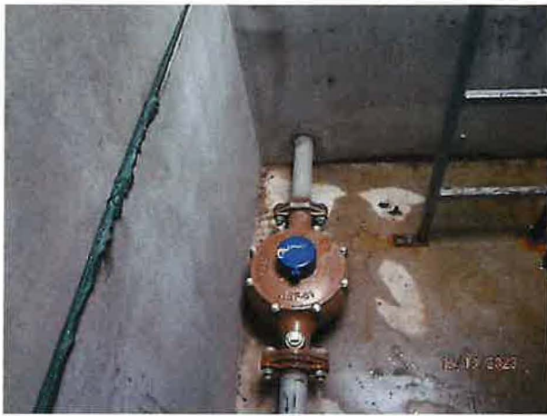
LINE COMING IN TO FLOW METER FROM STORAGE TANK (WITH PRESSURE PUMP) ABOVE AND PRESSURE TANK BELOW
