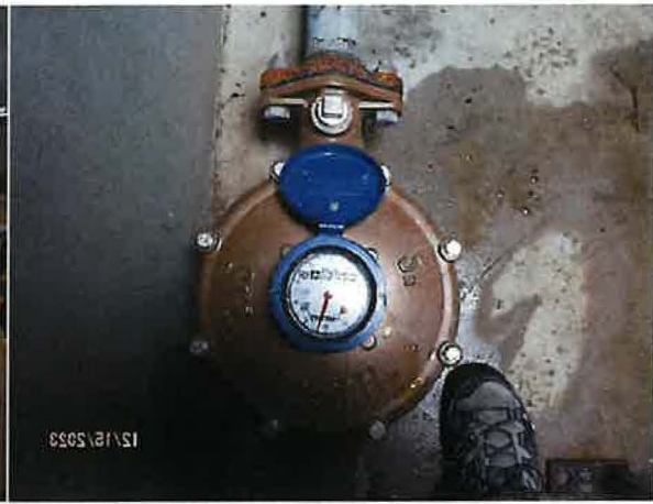
LINE COMING IN TO FLOW METER FROM STORAGE TANK (WITH PRESSURE PUMP) ABOVE AND PRESSURE TANK BELOW
