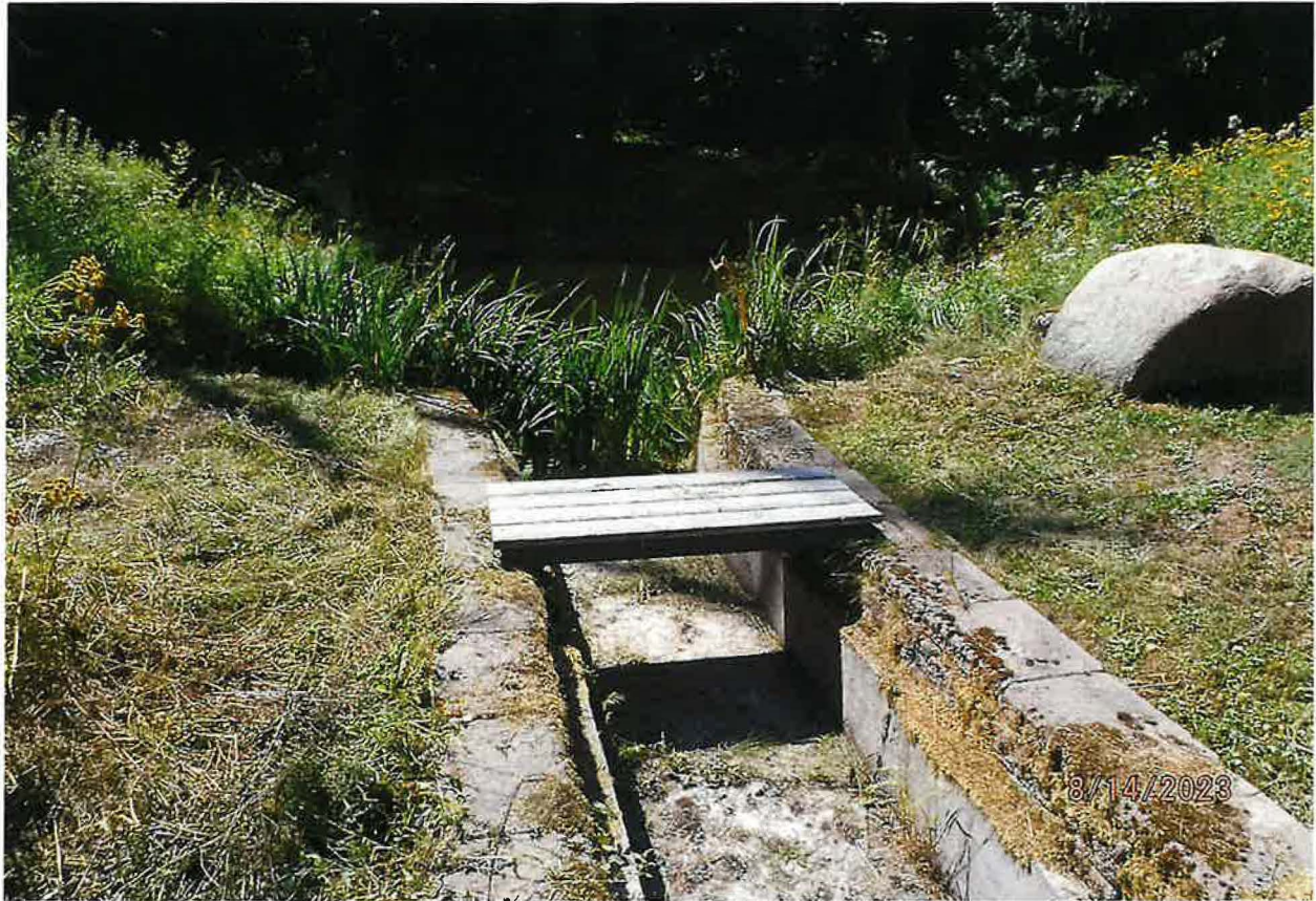
EASTERN STORAGE POND OVERFLOW DEVICE – CONCRETE RACEWAY TO SMALL WATERFALL
