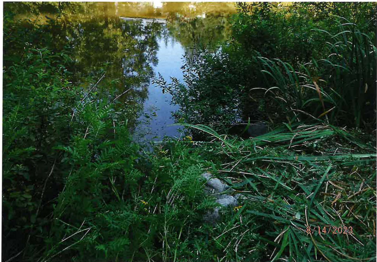
WESTERN STORAGE POND POD – EARTHEN DAM WITH ROCK OVERFLOW CHANNEL
