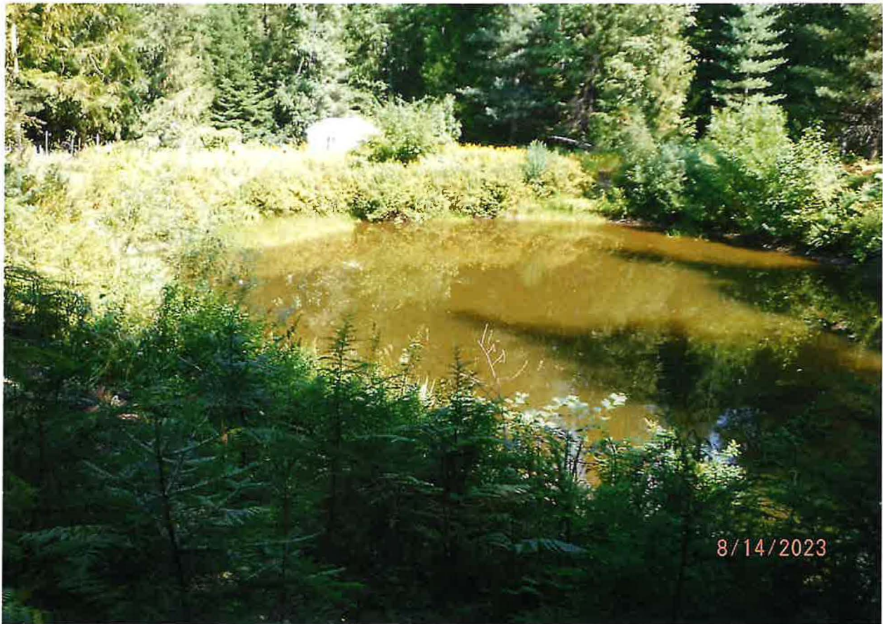
WESTERN STORAGE POND POU; POD EARTHEN DAM WITH OVERFLOW CHANNEL TO LOWER POND
