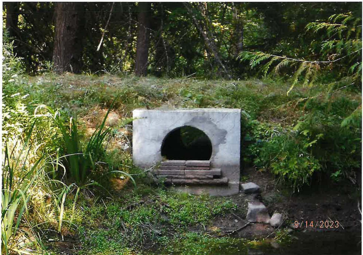
1 OF 2 OVERFLOW DEVICES – EASTERN POND, SECONDARY OVERFLOW CHANNEL
