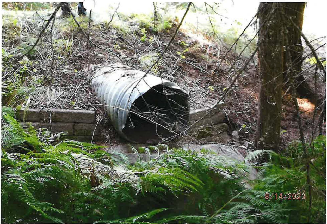
SECONDARY OVERFLOW CHANNEL FOR EMERGENCY PURPOSES – NE CORNER OF LOWER EASTERN POND
