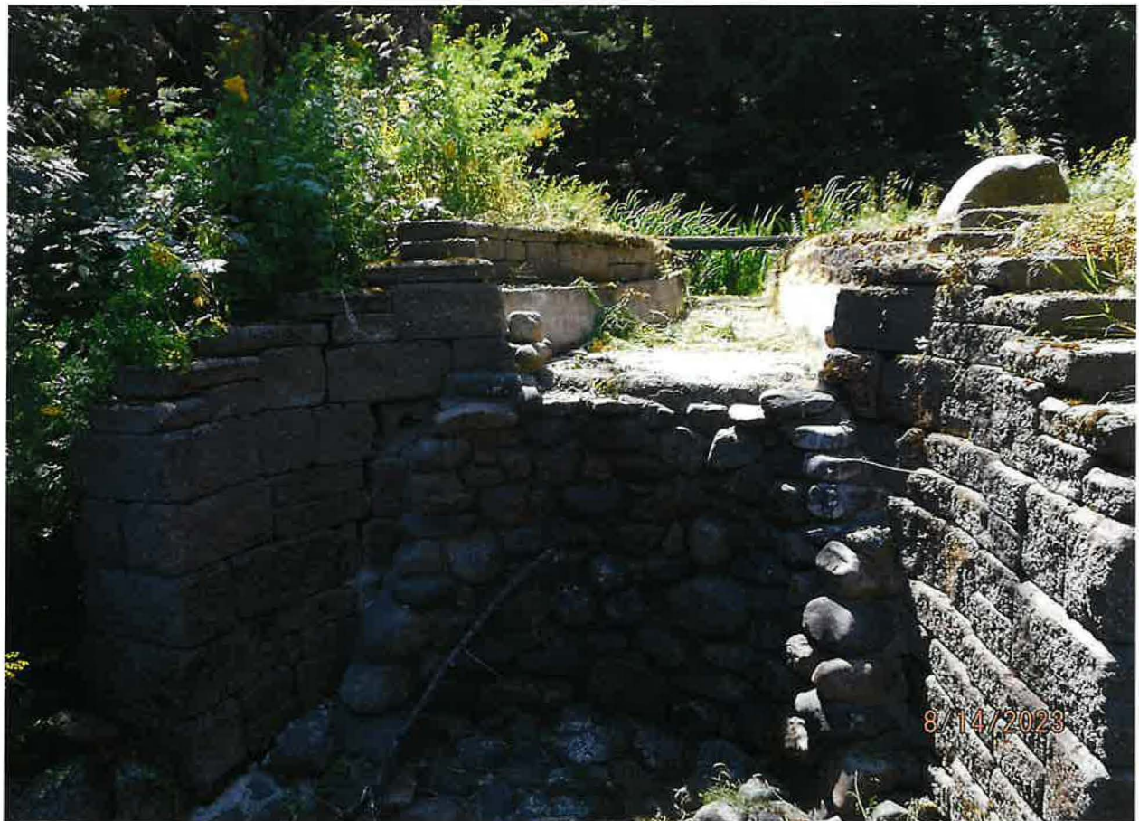
EASTERN STORAGE POND OVERFLOW DEVICE – CONCRETE RACEWAY TO SMALL WATERFALL
