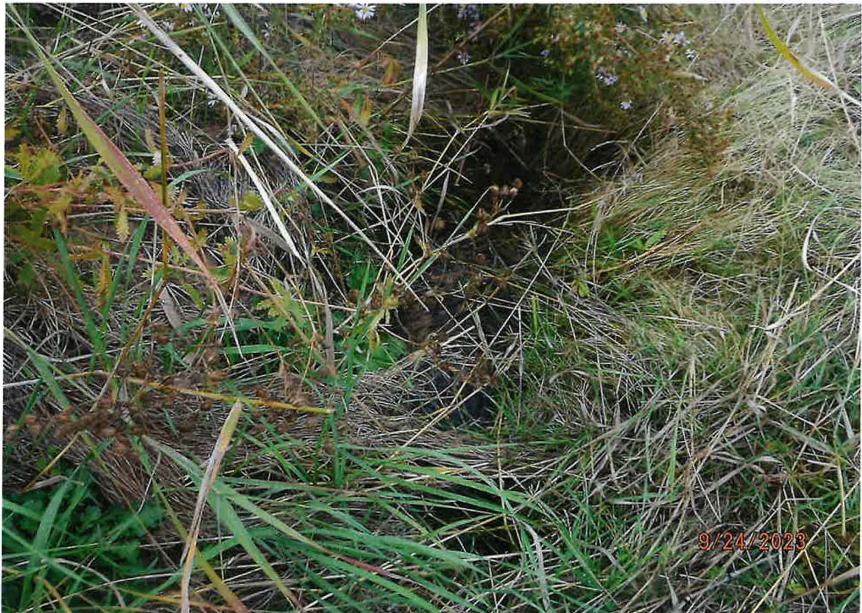
OVERFLOW PIPE LOCATED IN POND DISCHARGES TO DITCH
