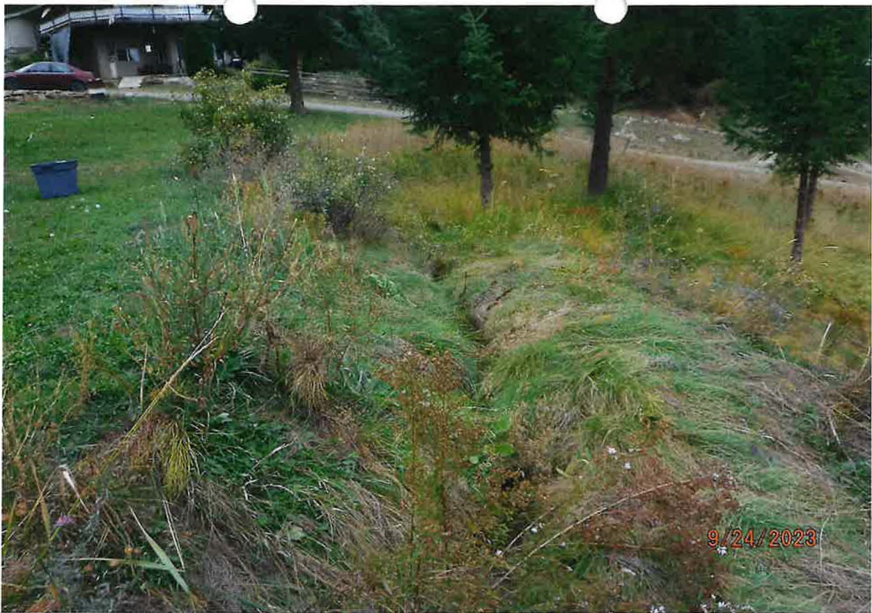
OVERFLOW DISCHARGE CHANNEL ROUTES WATER FROM THE UPPER POND DOWN A DITCH TO THE LOWER POND
