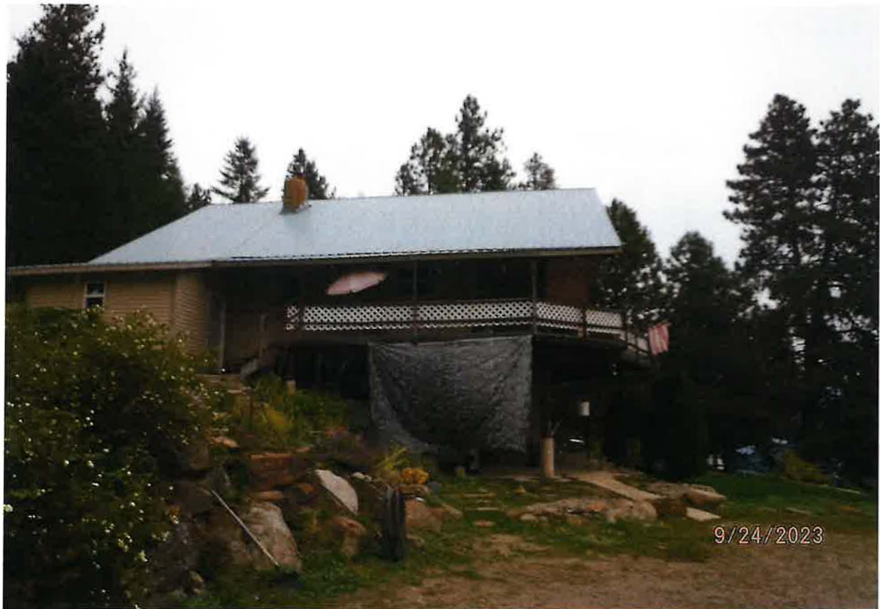
DOMESTIC POU – 1 HOME WITH 1 SHOP WHICH RECEIVES GRAVITY FLOW SPRING WATER
