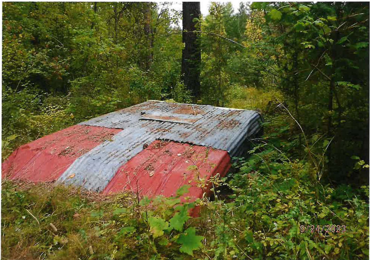
DIVERTING WORKS INCLUDE 550-GAL COVERED STORAGE RESERVOIR
