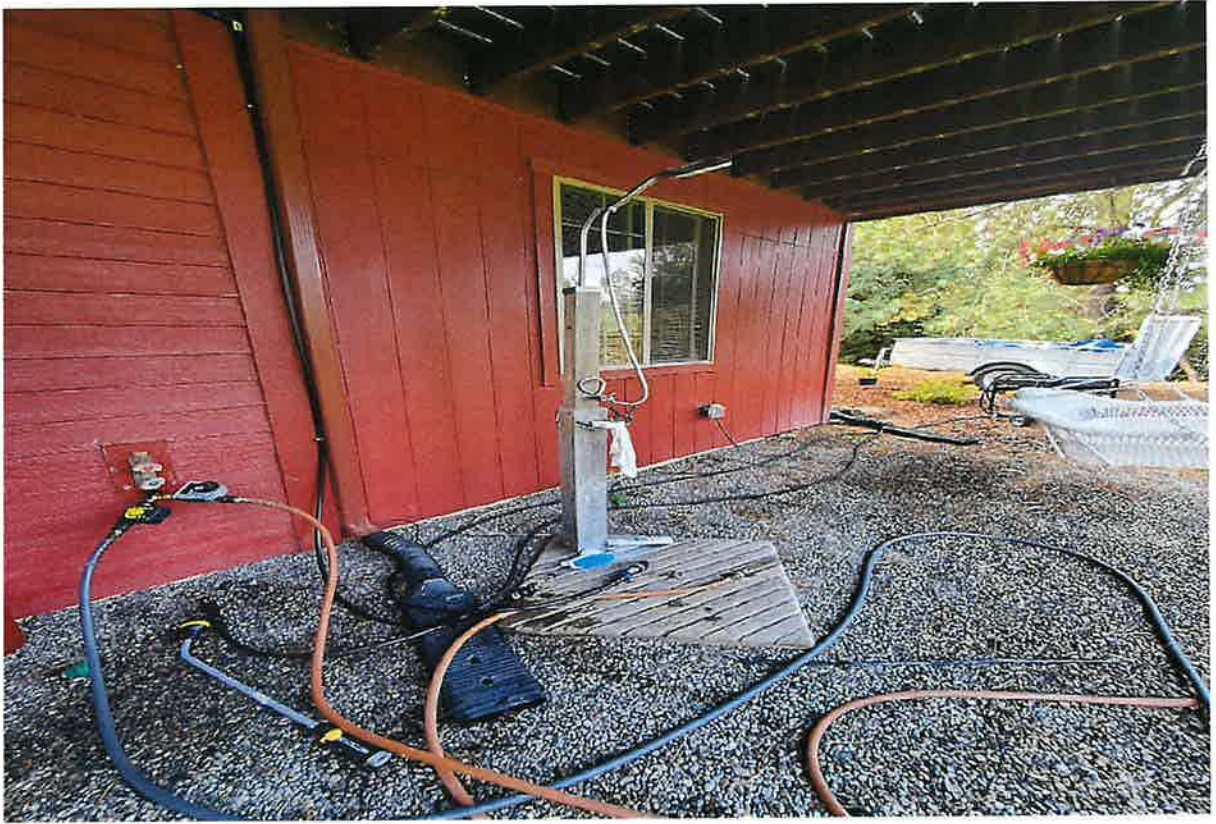
POU - IRRIGATION LINES INCLUDING DRIP SYSTEM FOR HANGING BASKETS
