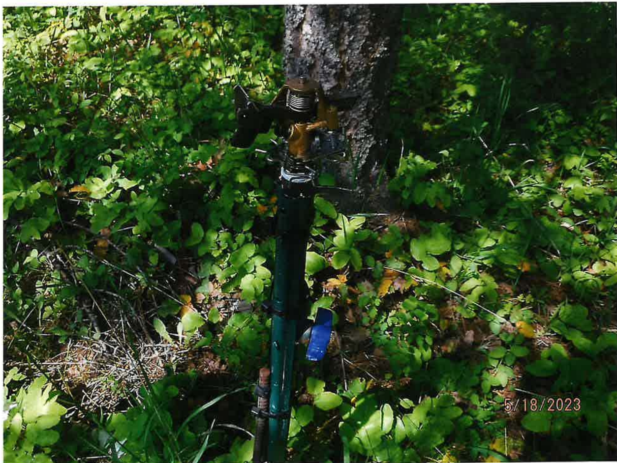
IRRIGATION POU – SPRINKLER RISER PIPE OFF MAIN TRUNK LINE
