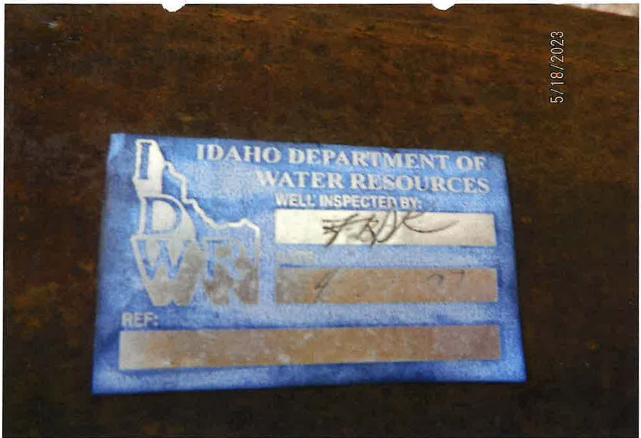
ILEGIBLE WELL INSPECTION TAG ON WELL CASING
