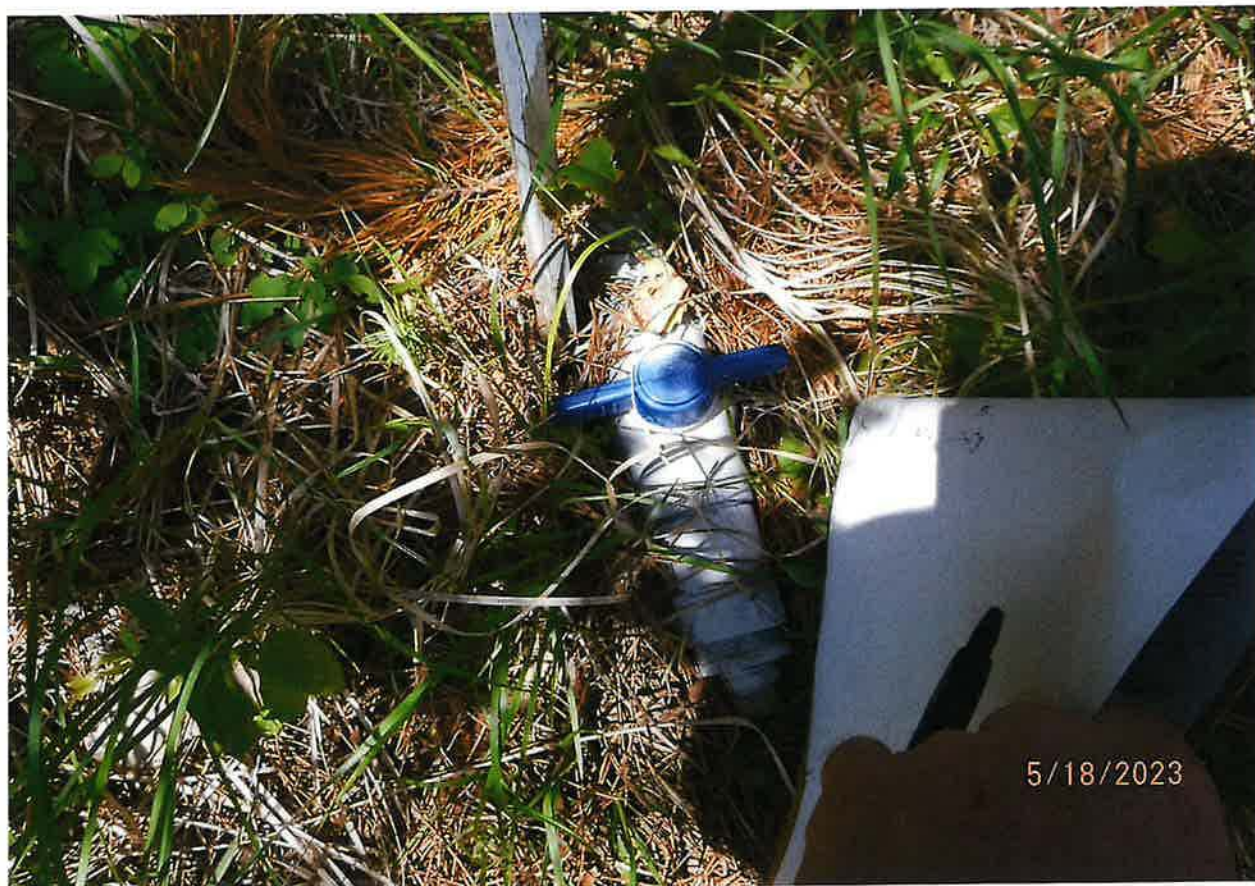
IRRIGATION RISER TO HOSE AND SPRINKLER
