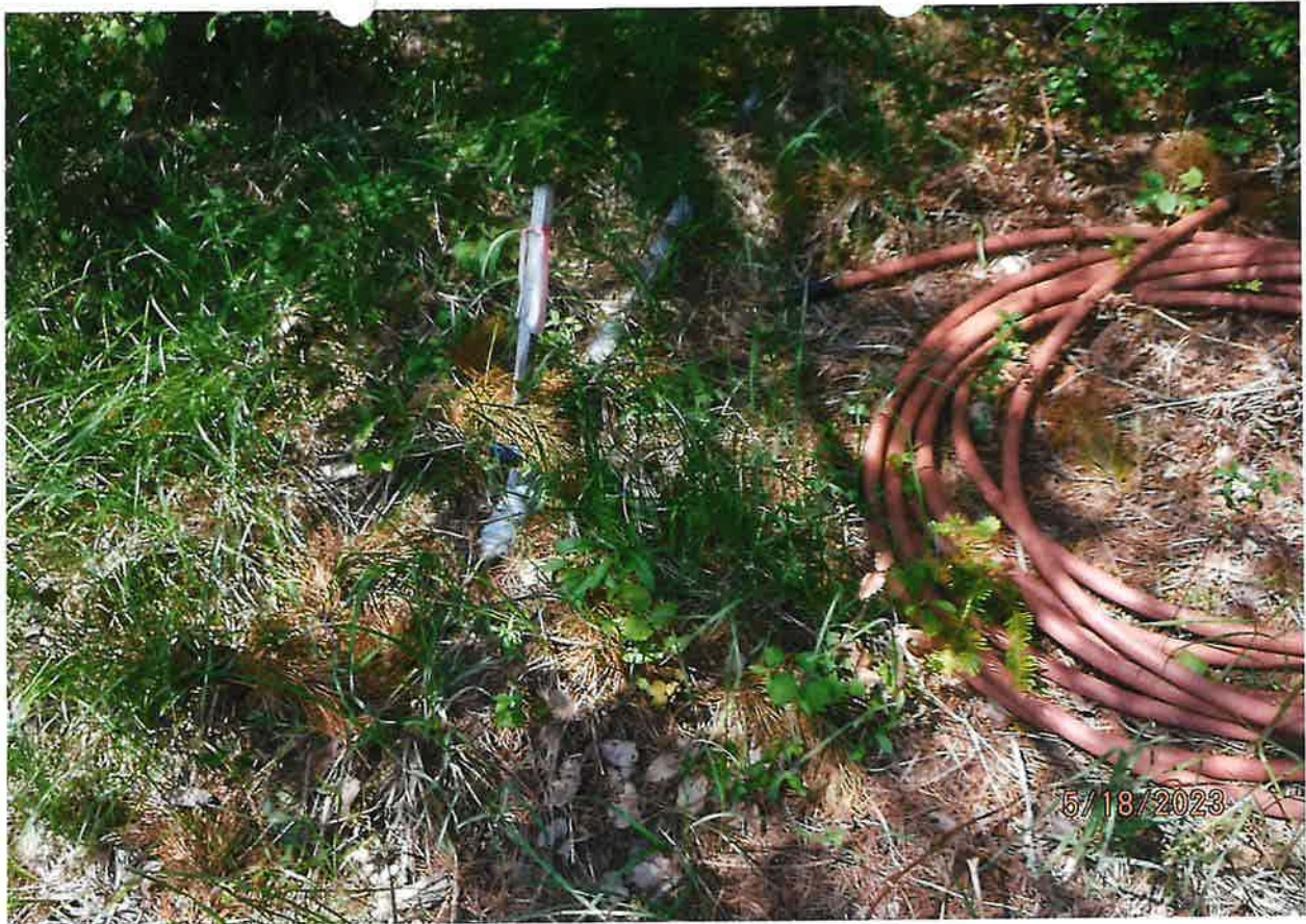
IRRIGATION RISER TO HOSE AND SPRINKLER
