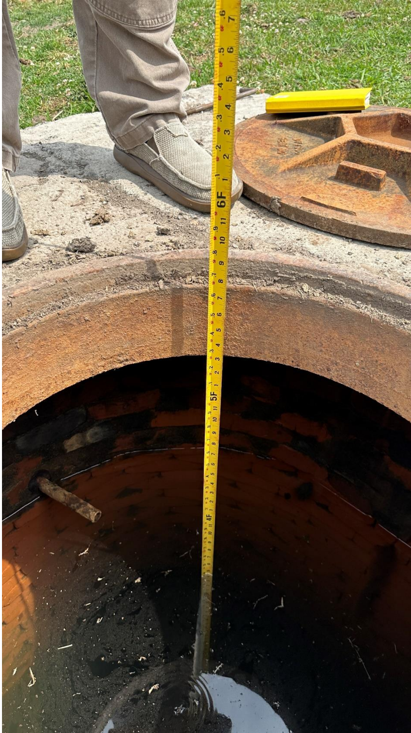
Photo 5: Measuring depth of well.
