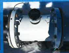
"No direct sunlight exposure" Unprotected Siemens 8000
