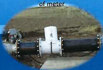
Bucket was cut-out to fit over curvature of meter
