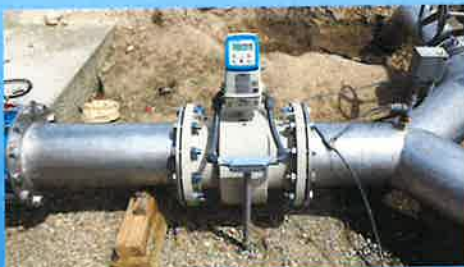
Siemens Sitrans F M Mag 8000, battery operated, external power not needed , internally grounded. Protect meter readout from weather.
