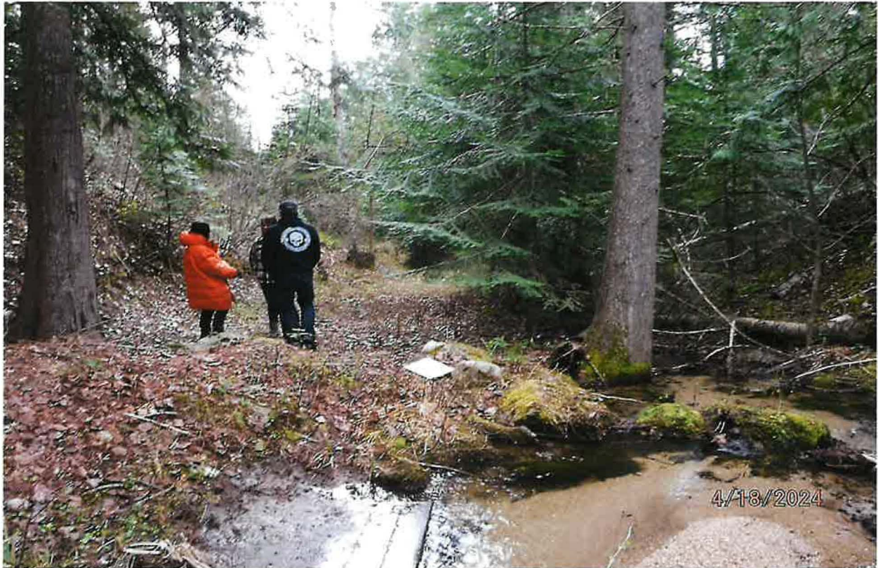
DIVERSION TO STORAGE – BURIED 2-INCH POLY PIPE ROUTED ALONG TRAIL DOWNGRADE TO STORAGE POND
