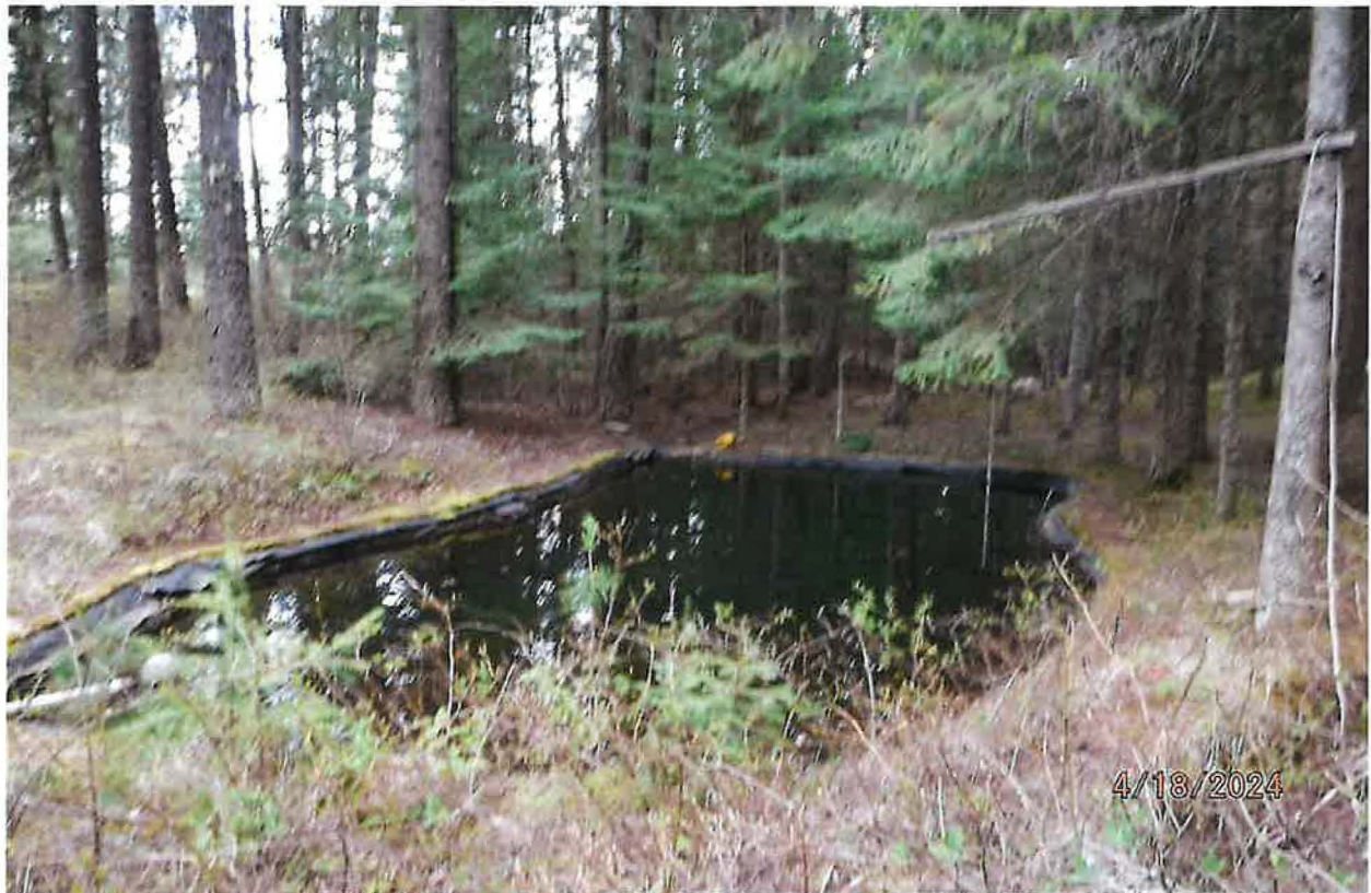
IRRIGATION STORAGE & FIRE PROTECTION STORAGE POU – LINED POND IN HEAVILY TREE CANOPY LOCATION ON PROPERTY
