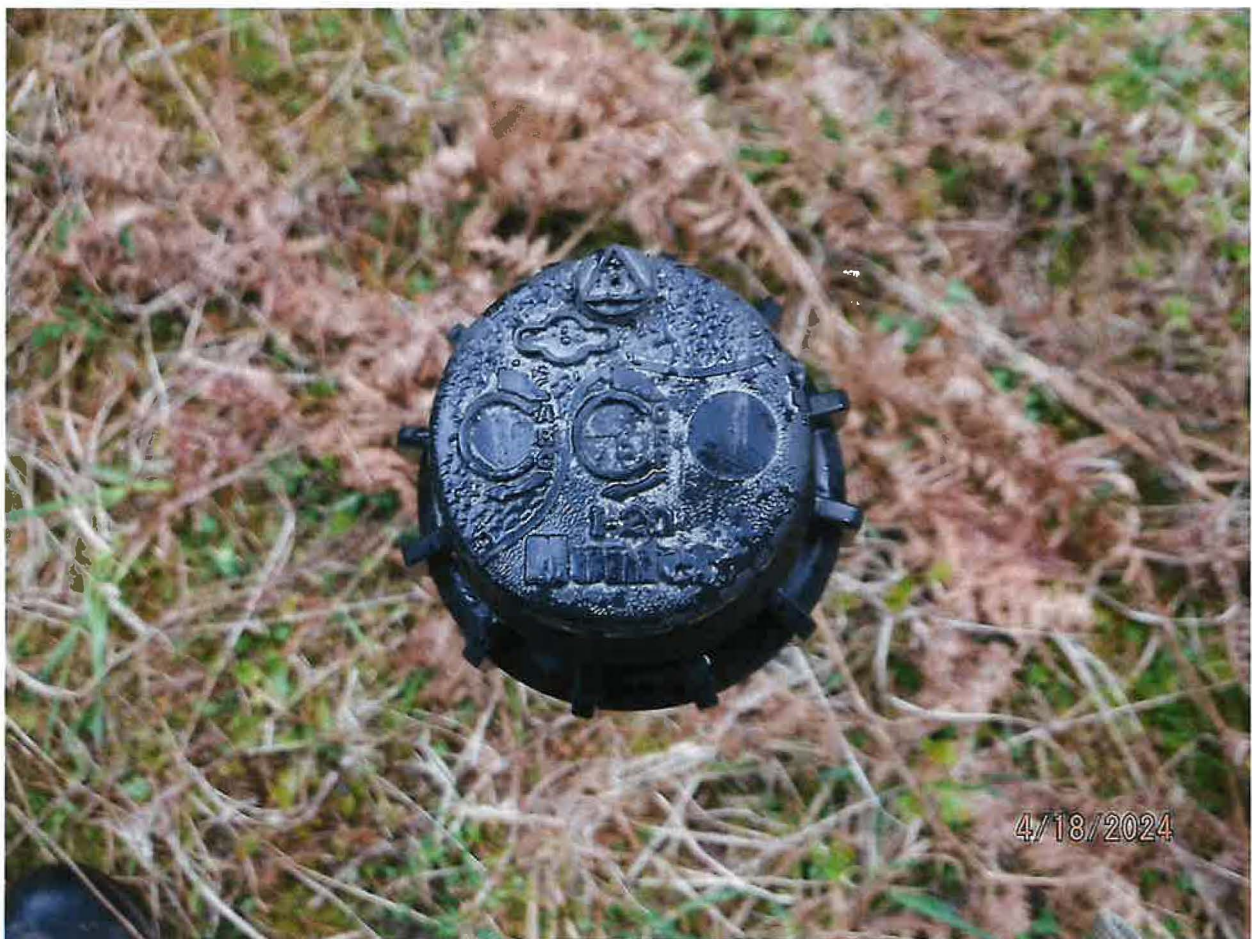
PRESSURIZED SPRINKLER – HUNTER MODEL (CENTER OF FRAME)
