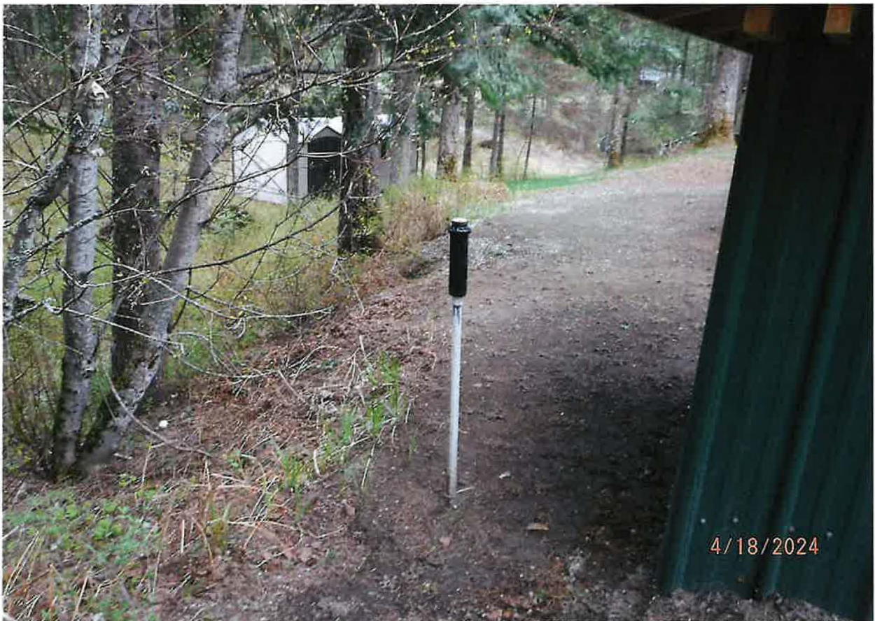
IRRIGATION RISER – USED TO WATER HILL SLOPE
