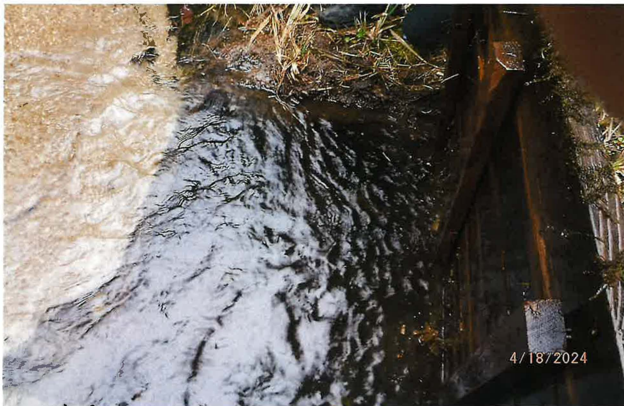
LID RAISED ON WOODEN COLLECTION BOX, WHITE POLY PIPE CENTER BOTTOM OF PHOTOGRAPH (SLIGHTLY WASHED OUT IN IMAGE FROM REFLECTION)
