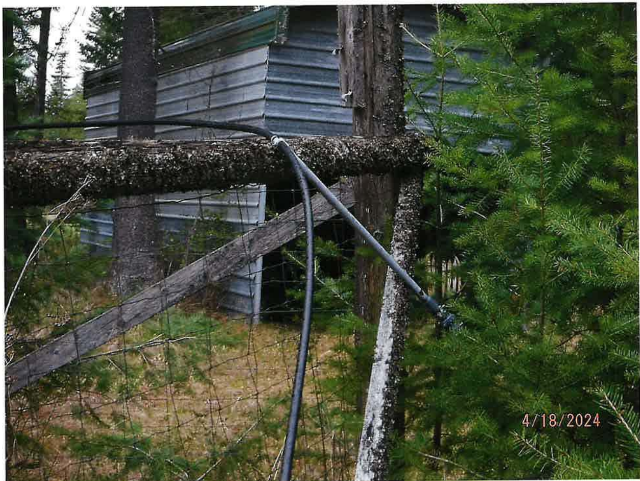
IRRIGATION FROM STORAGE – SPRINKLER RISER ON GARDEN POST USED TO WATER TREE PLOT
