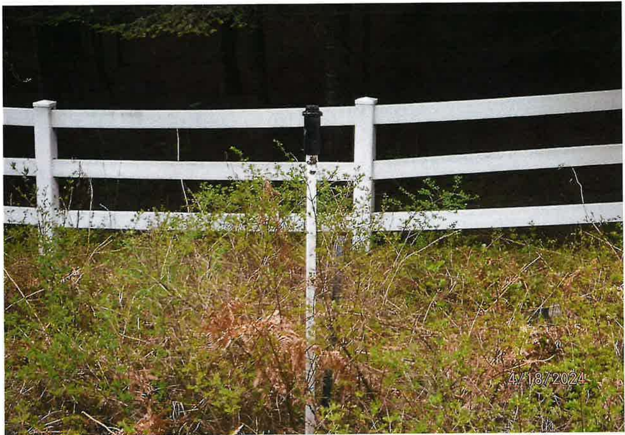
IRRIGATION FROM STORAGE – RISER PIPE WITH HUNTER 360 DEGREE PRESSURIZED SPRINKLER HEAD
