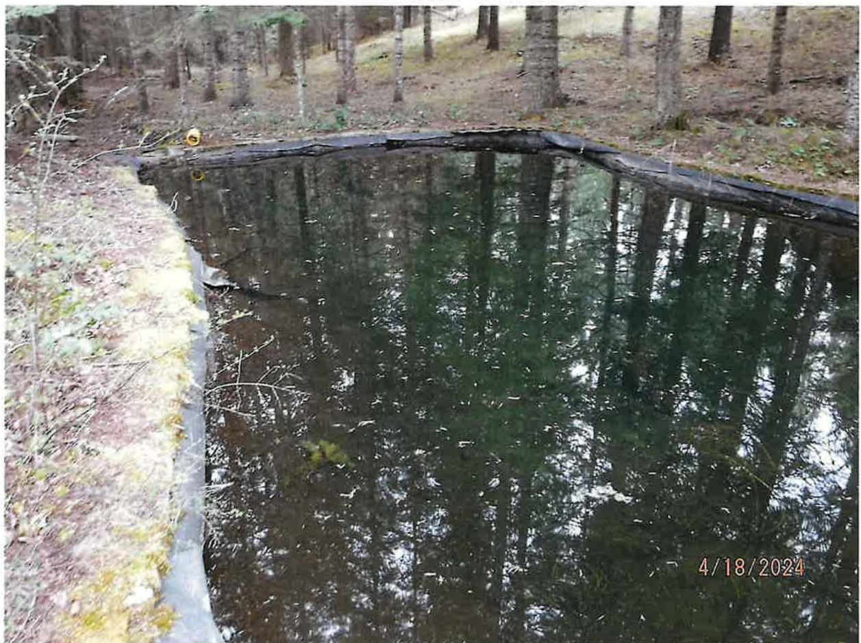
IRRIGATION STORAGE & FIRE PROTECTION STORAGE POU – LINED POND IN HEAVILY TREE CANOPY LOCATION ON PROPERTY
