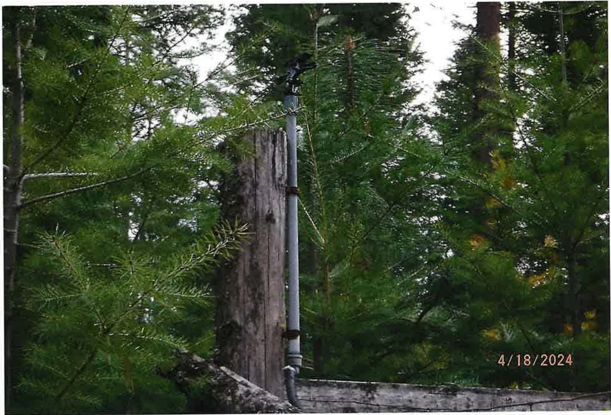
IRRIGATION FROM STORAGE – SPRINKLER RISER ON GARDEN POST USED TO WATER TREE PLOT
