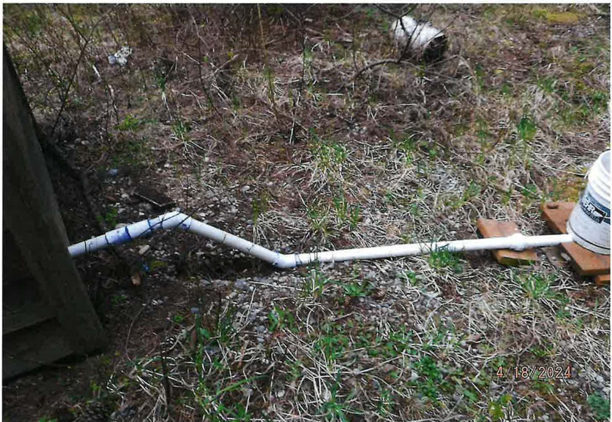
FROM STORAGE PIPELINE
