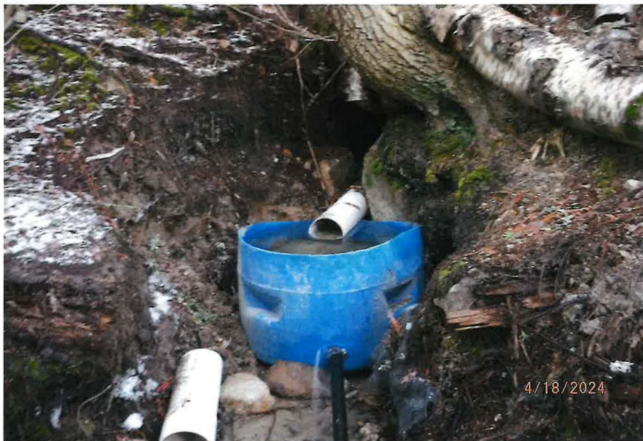
POD – SPRING WITH PVC PIPE TO CONTAINMENT DEVICE
