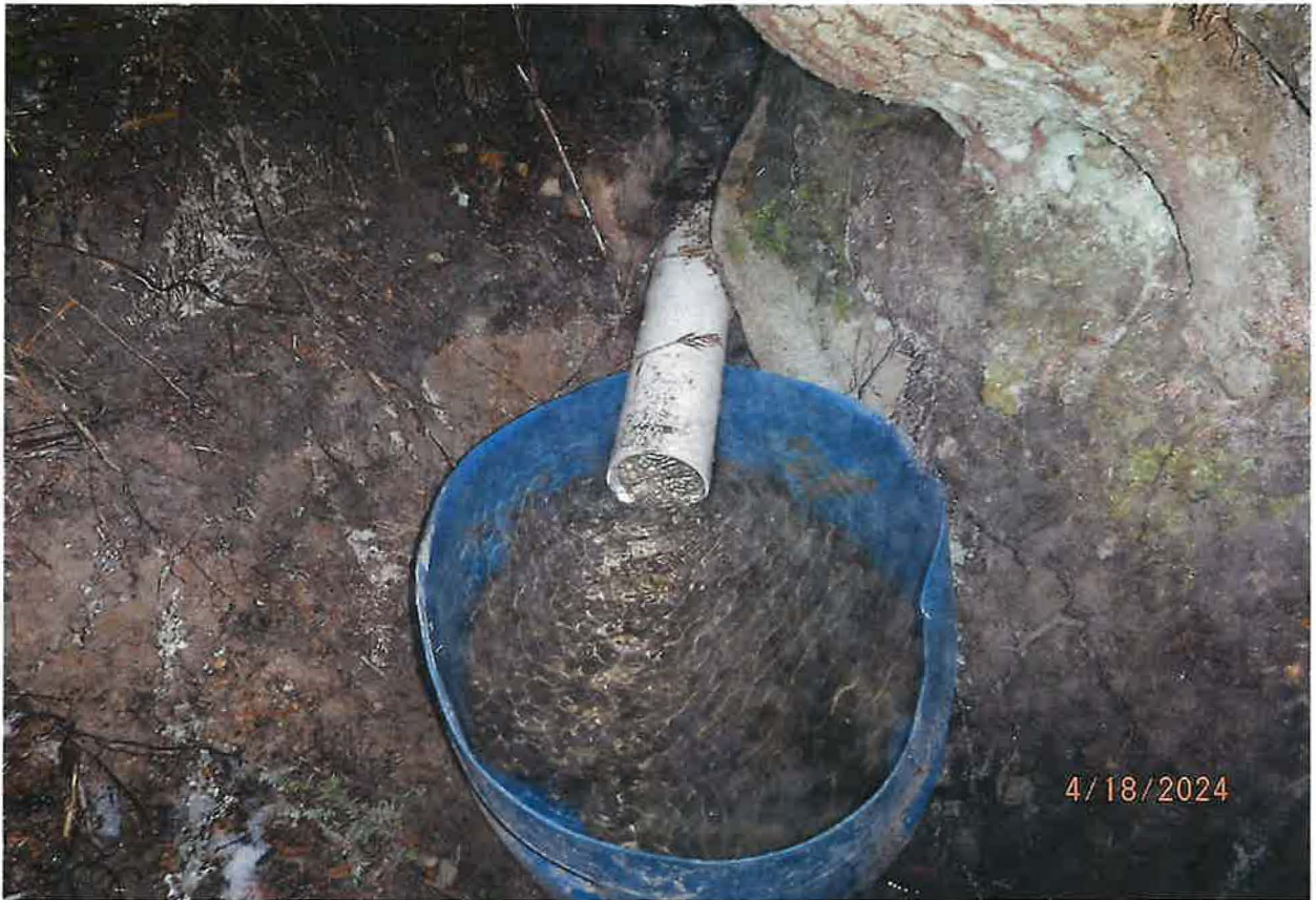
POD – SPRING COLLECTION POINT ROUTES TO \frac{3}{4} " POLY PIPE RUNNING DOWN SLOPE TO STORAGE TANK PRIOR TO WATER USE FOR DOMESTIC PURPOSES.
