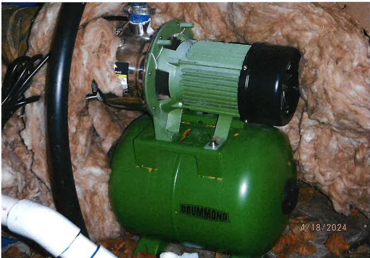
DRUMMOND 1 HP STAINLESS STEEL SHALLOW WELL PUMP AND TANK WITH PRESSURE CONTROL SWITCH – 950 GPH (15.8 GPM) PUMP CAPACITY
