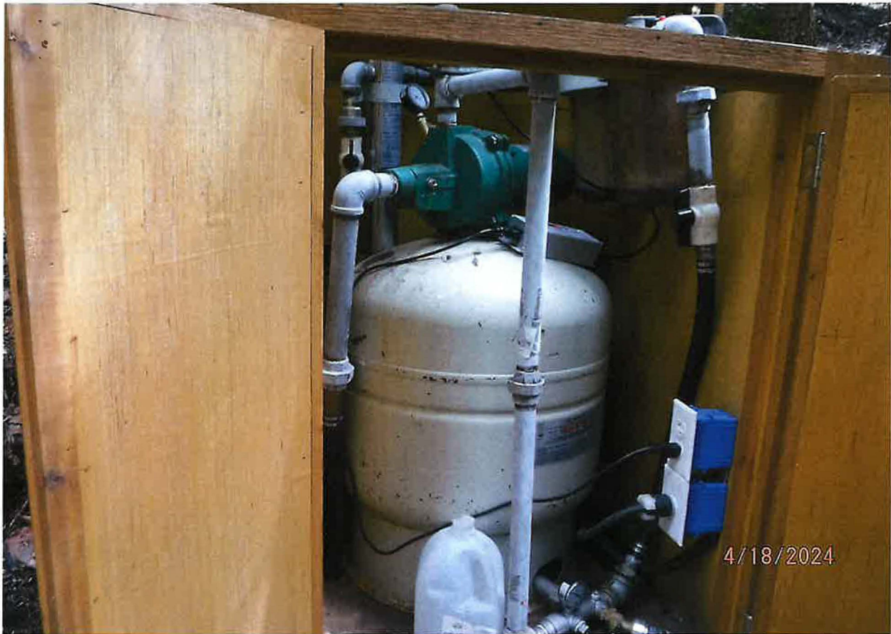
DIVERTING WORKS – LOCATED ALONG THE STREAM BANK AT POD
