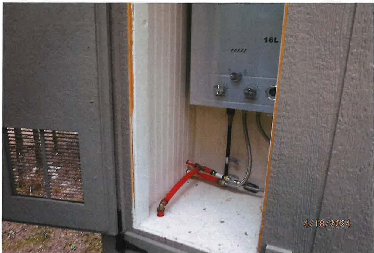
ON-DEMAND HOT WATER HEATER INSTALLED FOR RESTROOM
