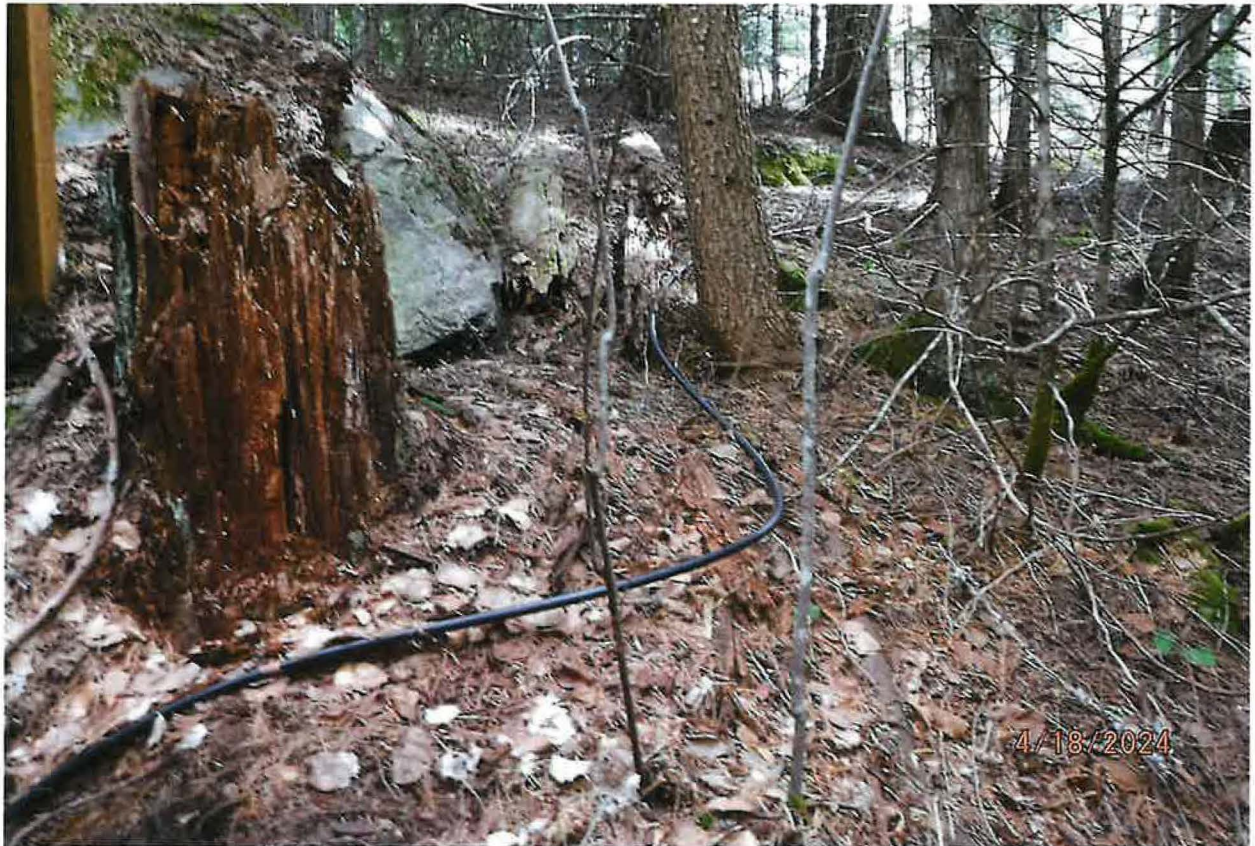
3/4" DISCHARGE PIPE FROM PUMP TO POU FOR WATER USE
