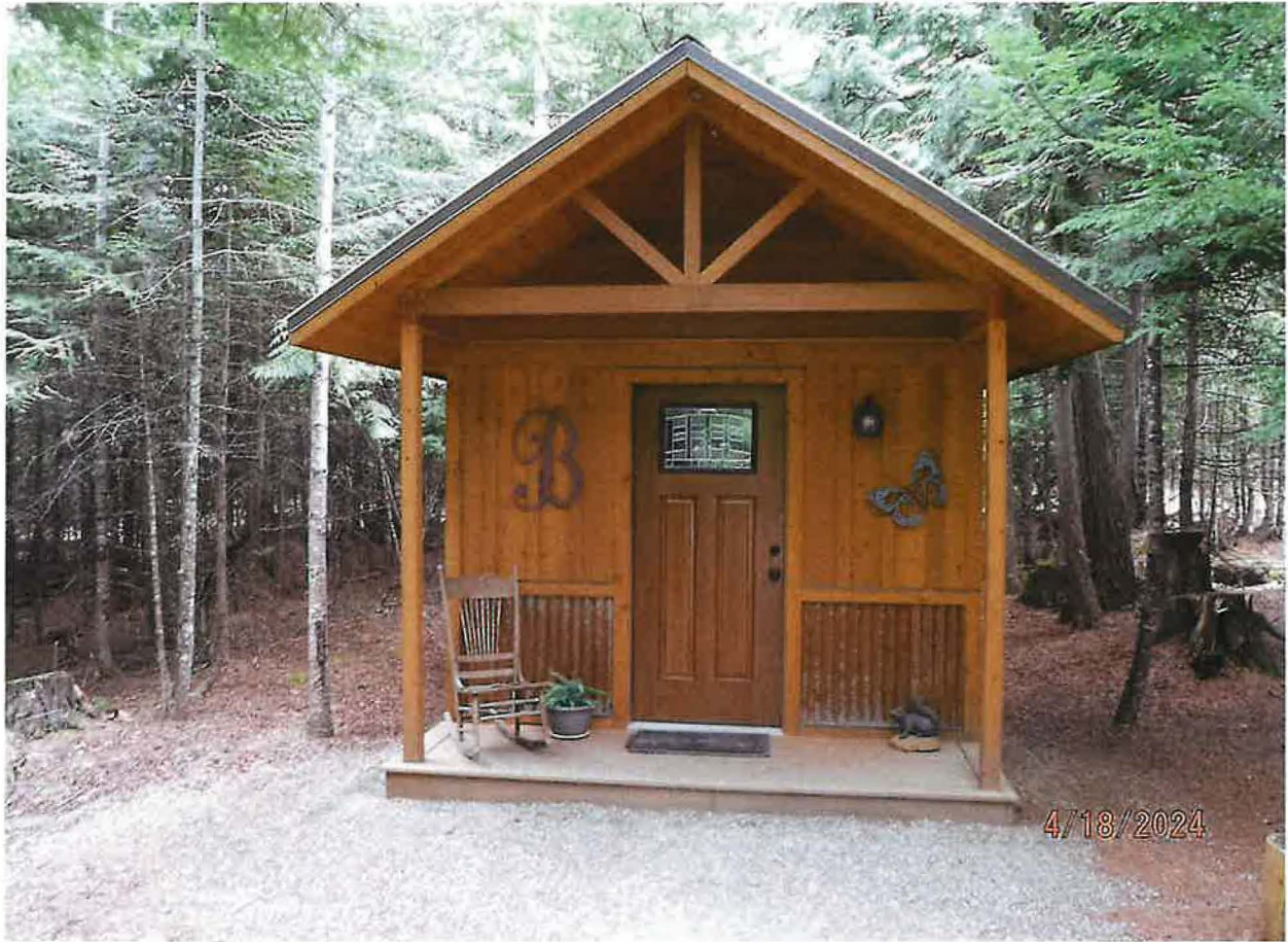
DRY ADU NO WATER SERVICES TO UNIT – EXTERNAL RESTROOM USED FOR GUESTS THAT USE THIS DRY ADU
