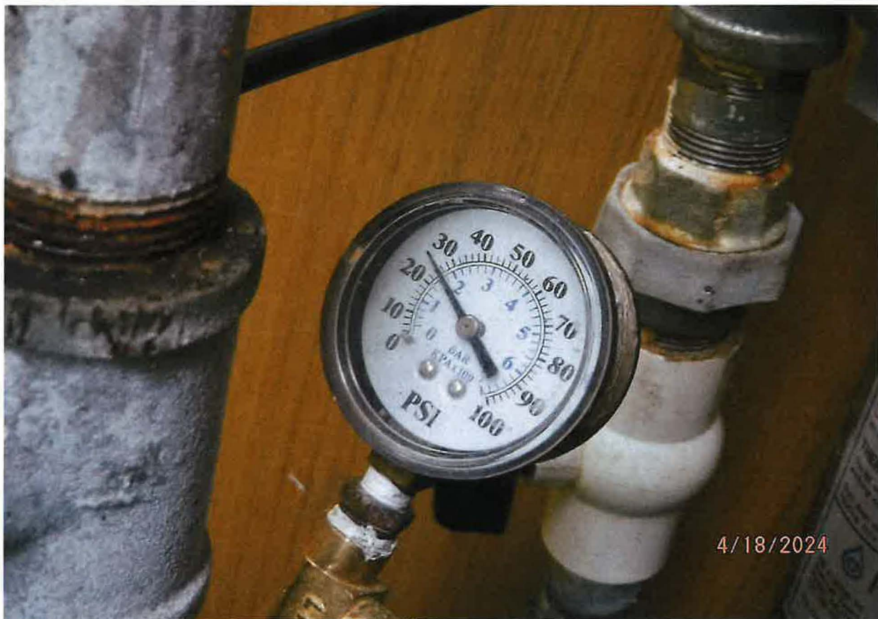
SYSTEM PRESSURE POT STATICALLY HOLDS AT 25 PSI
