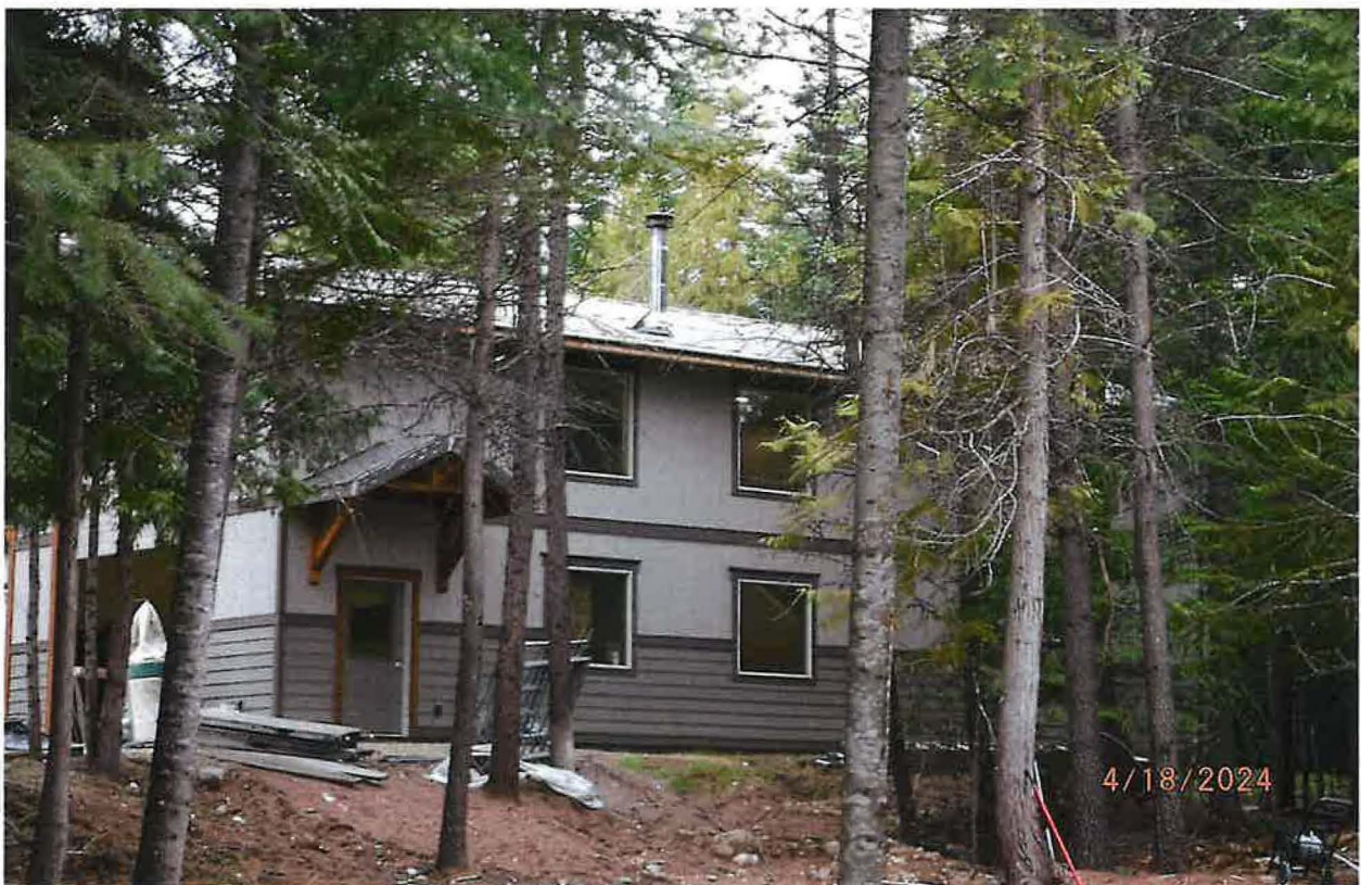
DOMESTIC POU – TWO STORY SHOP WITH FULL SERVICES (WASHER/SHOWER/BATHROOMS/SINKS)
