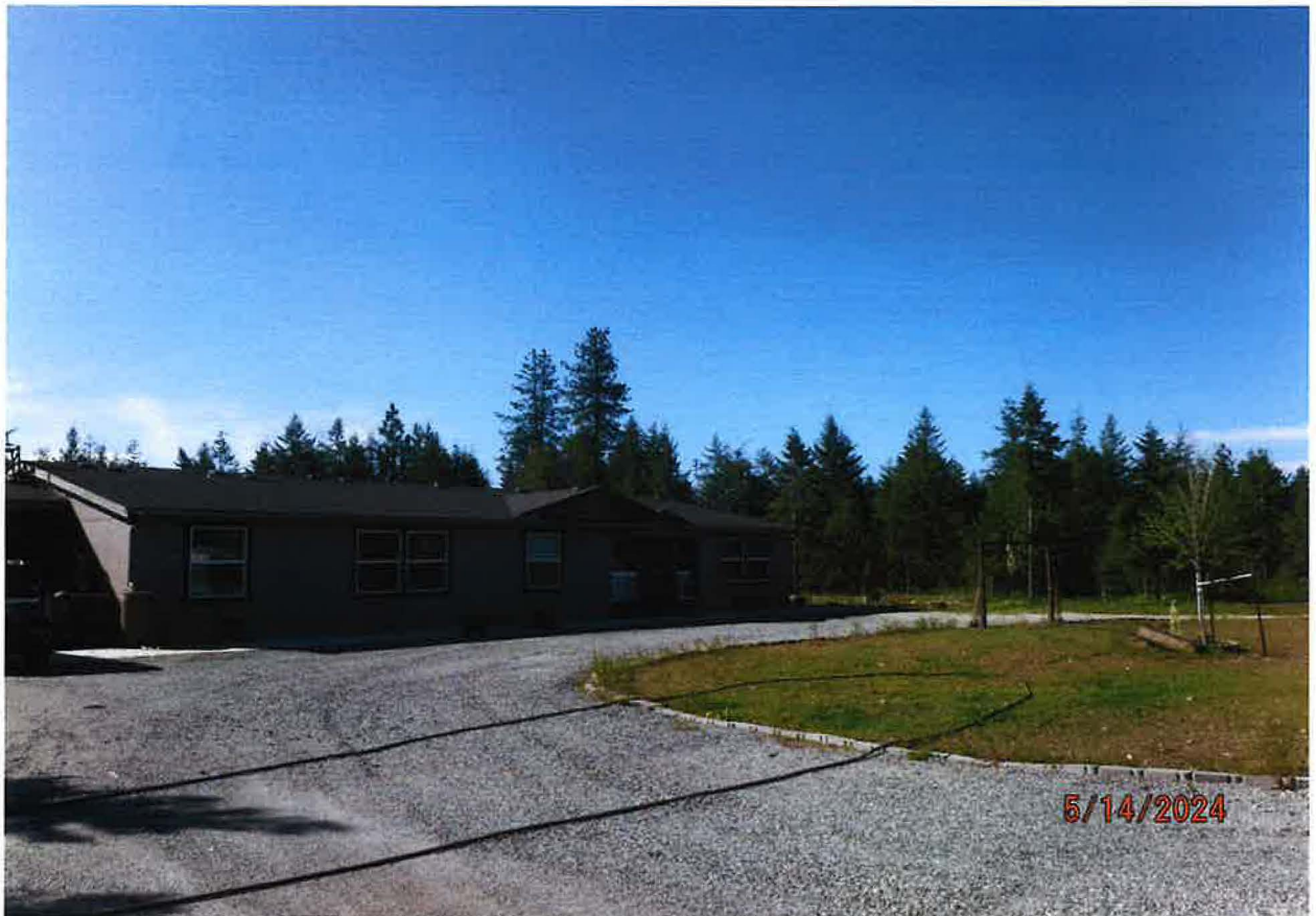
IRRIGATION POU – LOT 4
