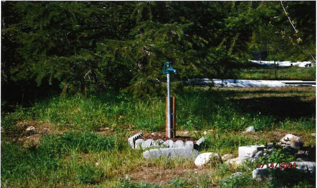
IRRIGATION POU – LOT 4
