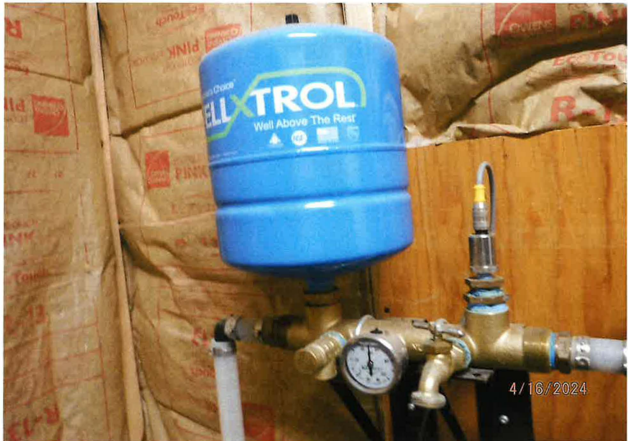
IRRIGATION FROM STORAGE SYSTEM STATIC PRESSURE 50 PSI
