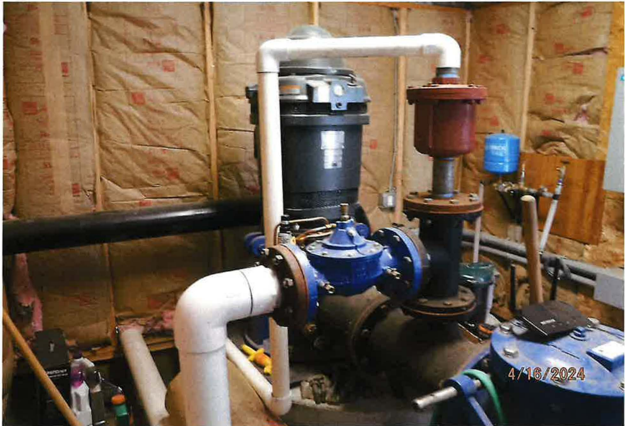
DIVERTING WORKS – INCLUDE A 75 HP 460V 3 PH US MOTOR, 1500 GPM FLOWISE LINE SHAFT TURBINE PUMP USED FOR FIRE PROTECTION PURPOSES
