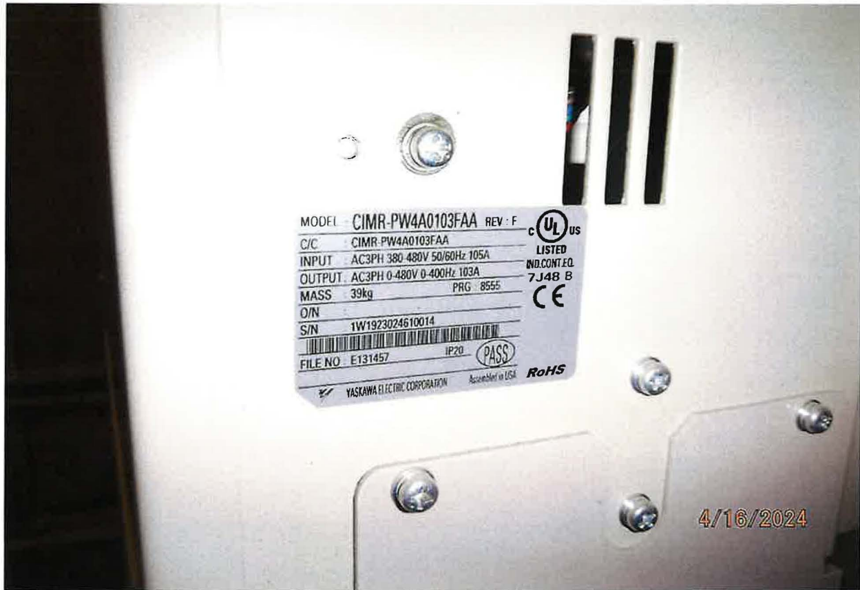
IRRIGATION FROM STORAGE PUMP CONTROL S/N 1W1923024610014
