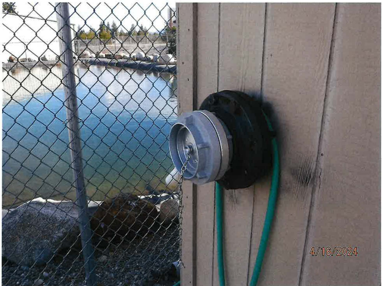
FIRE PROTECTION POU – MAIN FIRE TRUCK FILL PORT CONNECTS AT EXTERIOR OF PUMP STATION
