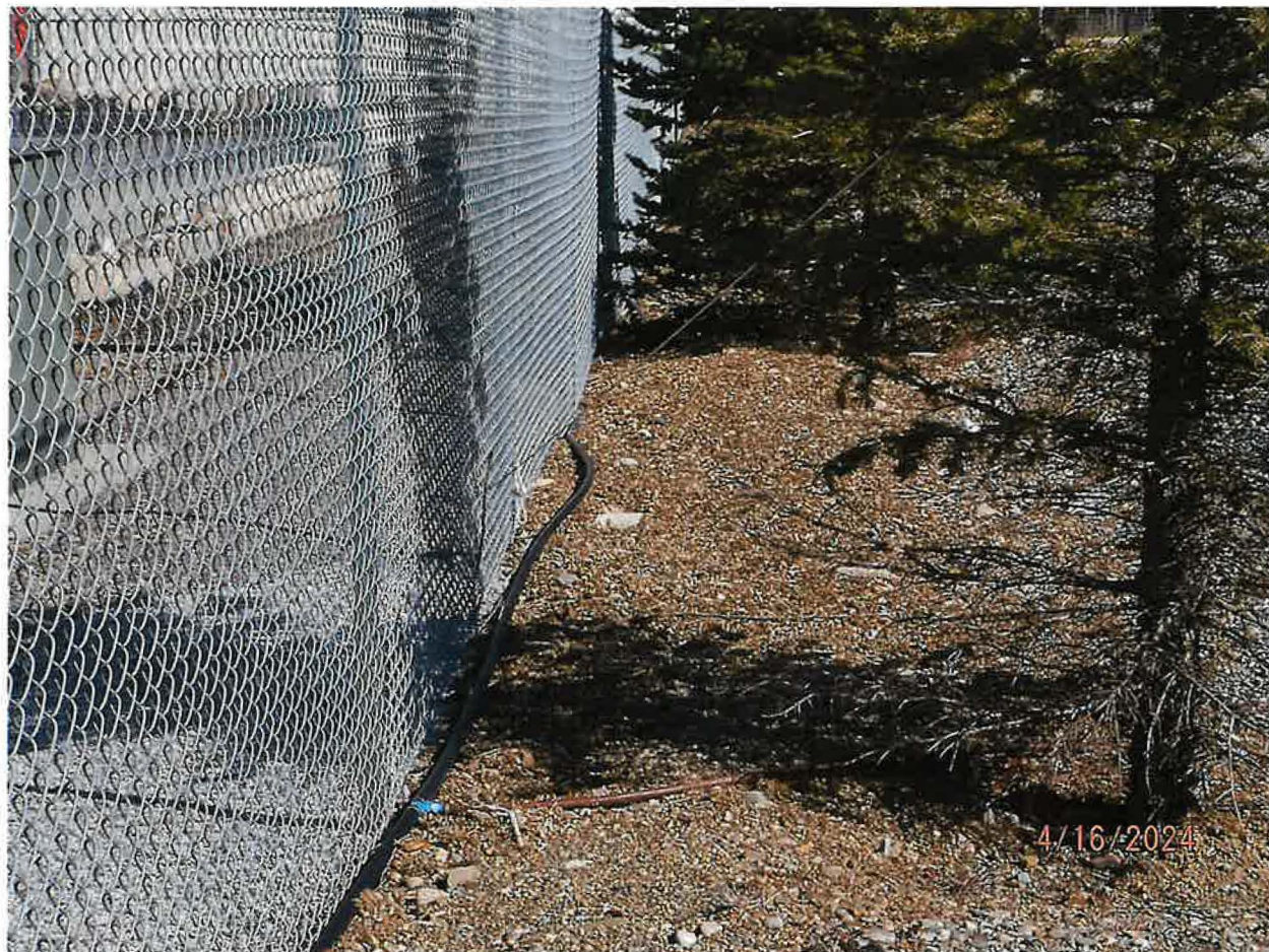
IRRIGATION FROM STORAGE – 1-INCH POLY PIPELINE ROUTING EAST FROM PUMP STATION TO FENCE LINE, ROUTING NORTH/SOUTH ALONG EAST FENCE LINE WATERING TREE ROW
