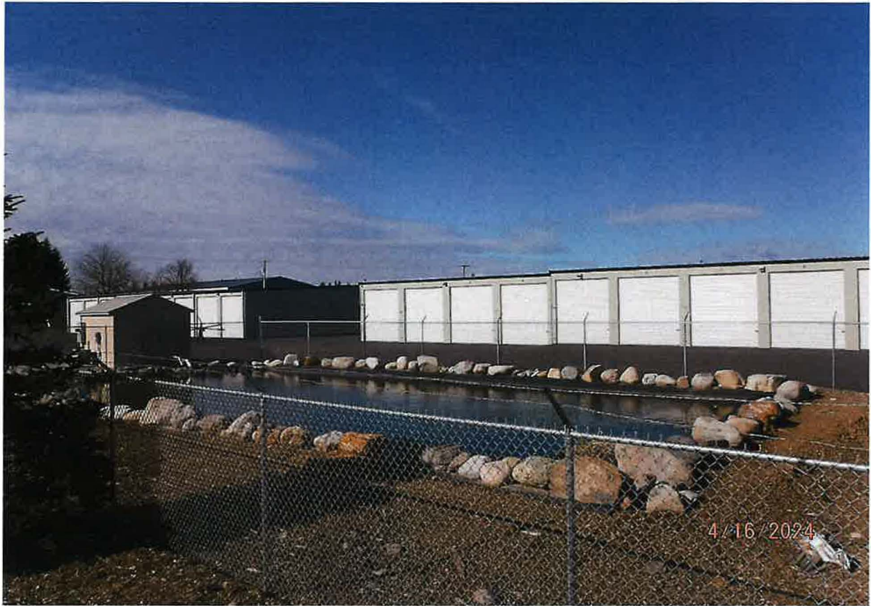
POU – FIRE PROTECTION STORAGE & IRRIGATION STORAGE LINED POND
