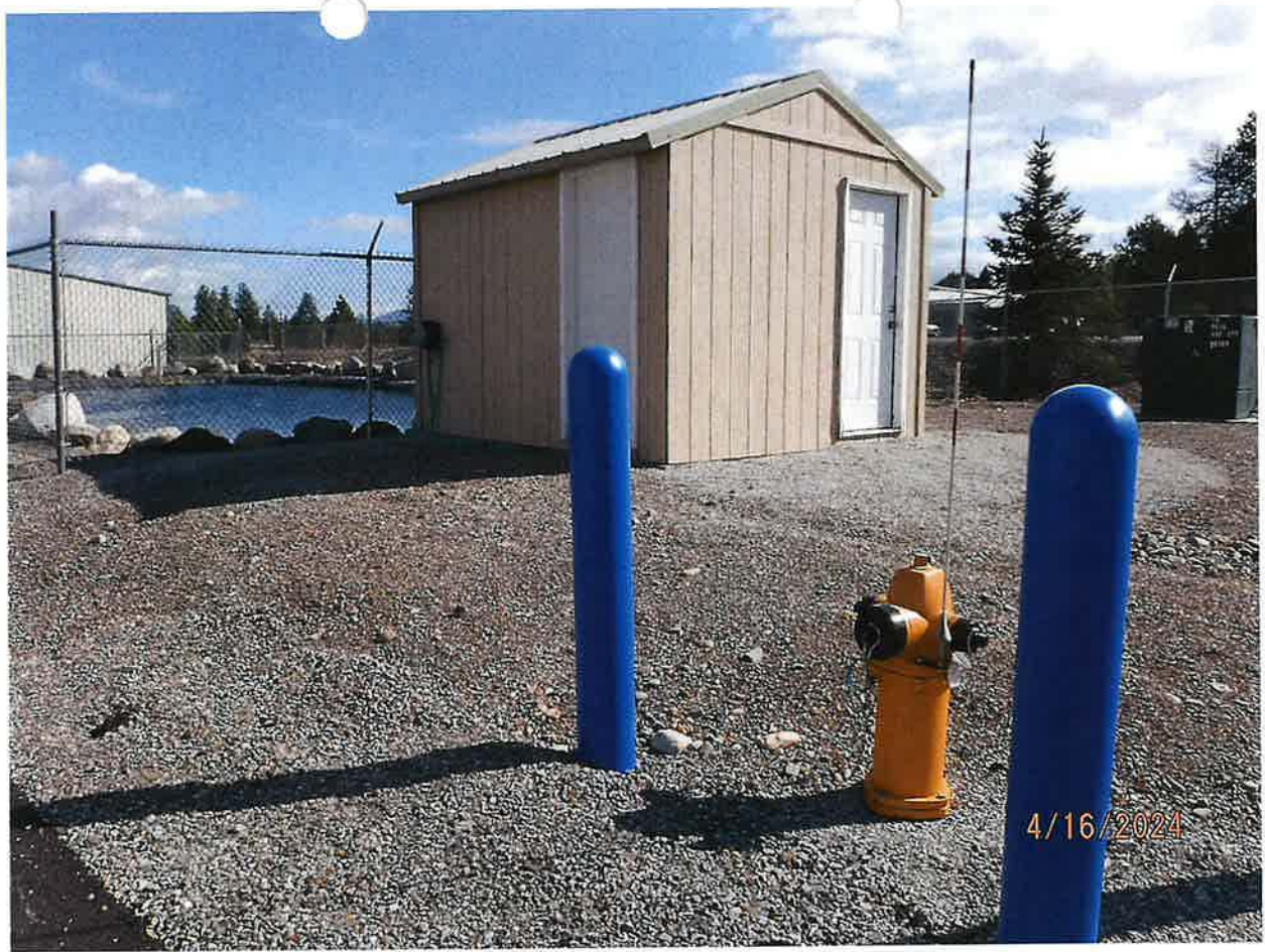
FIRE PROTECTION POU – TWO DEDICATED FIRE HYDRANTS POSITIONED IN STORAGE UNIT FACILITY
