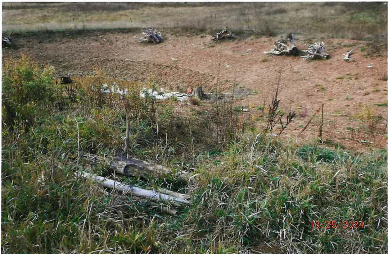
POU – NORTHERN FIRE PROTECTION & AESTHETIC STORAGE POND WITH UNNAMED STREAM INFLOW CHANNEL
