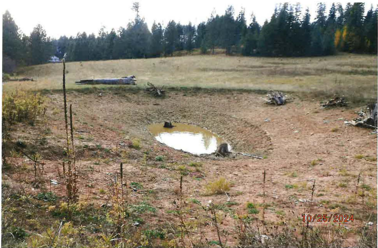
POU & POD – NORTHERN STORAGE POND EXCAVATED ENTIRELY BELOW THE NORMAL GROUND ELEVATION WITH MINOR OVERFLOW EARTHEN CHANNEL ALLOWING INTERMITTENT STREAM TO SPILL FROM POND
