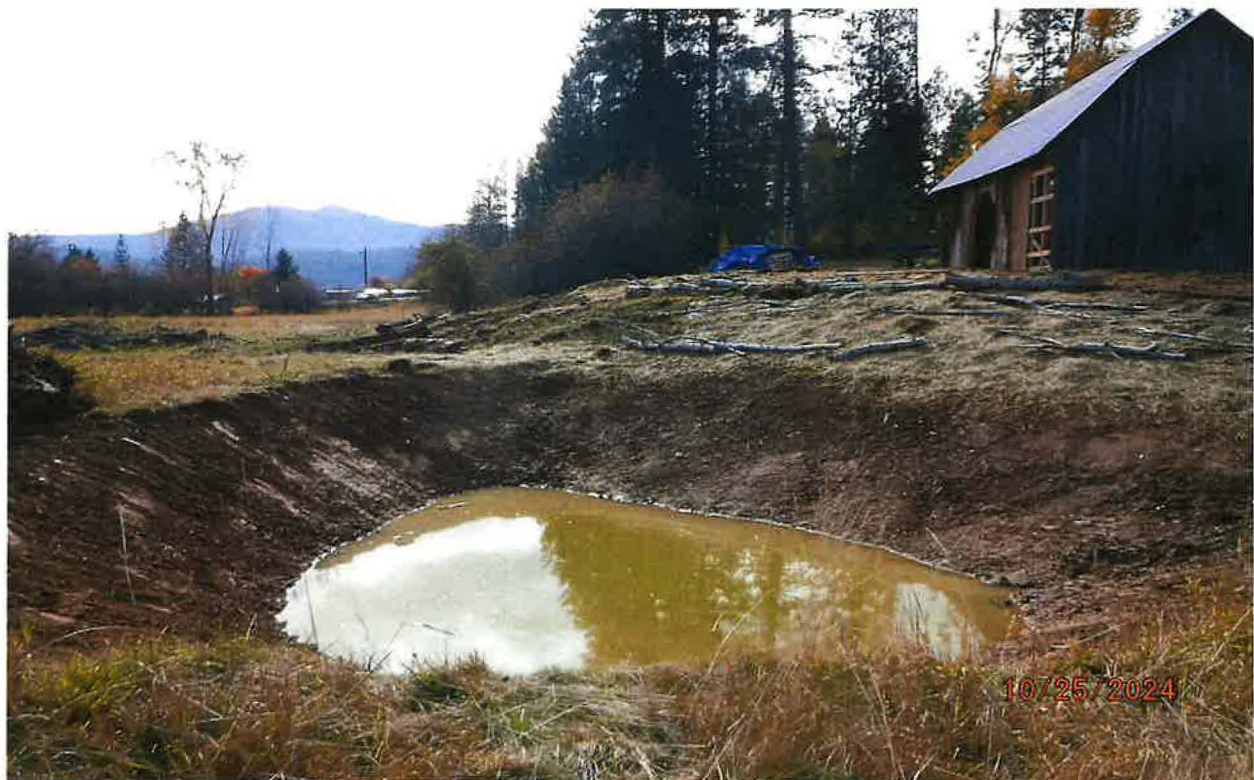
POU – SOUTHERN STORAGE POND USED FOR FIRE PROTECTION AND AESTHETIC USES.
