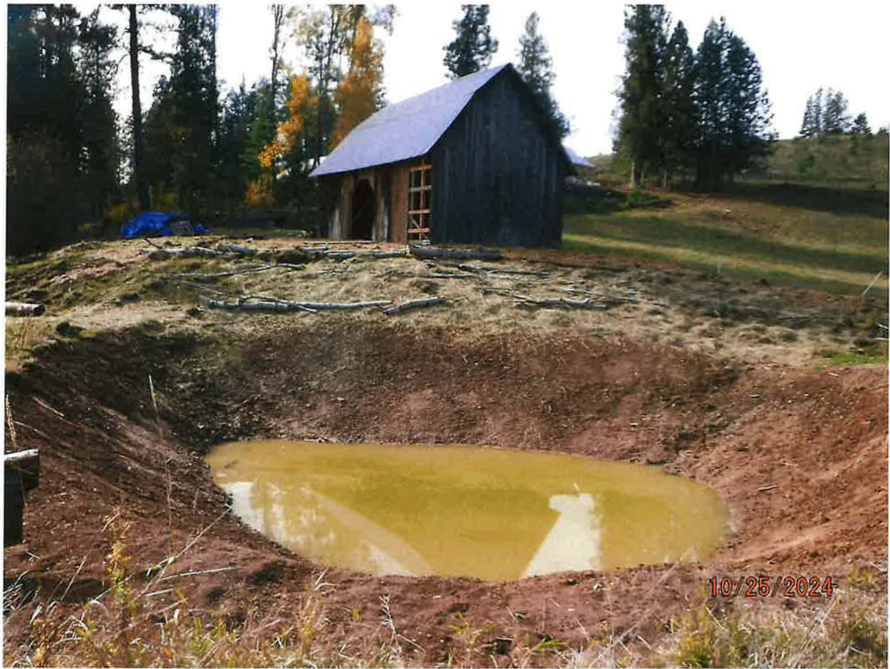
POD – SOUTHERN POND EXCAVATED ENTIRELY BELOW NORMAL GROUND ELEVATION WITH EARTHEN SPILL CHANNEL ADDED TO ALLOW INTERMITTENT STREAM FLOW TO SPILL FROM POND
