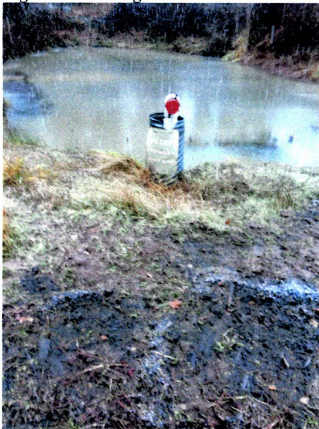
Figure 9: Pond Hydrant
