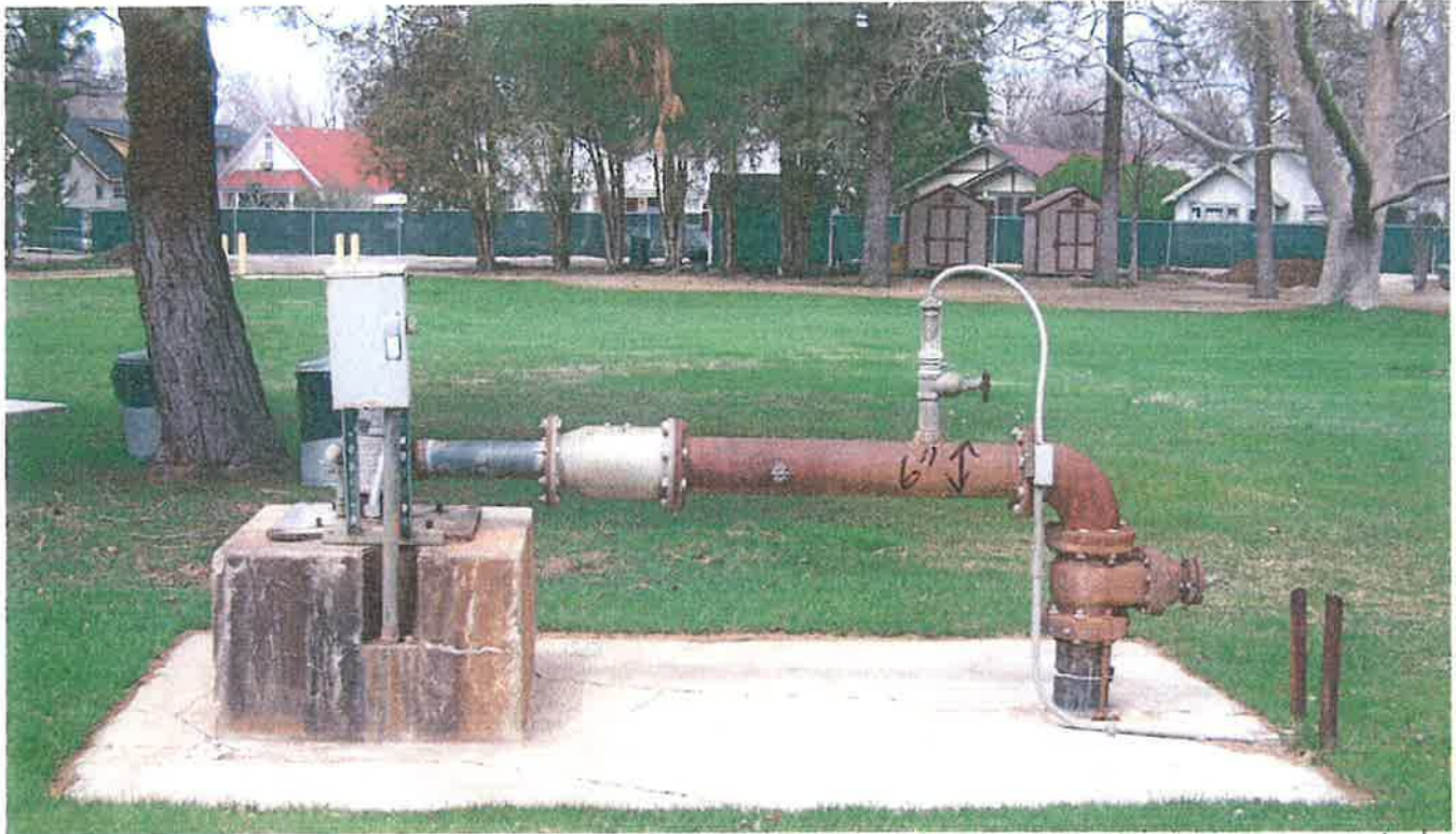
A63-5220 New well #1 Veterans Administration Medical Center 4/7/2006 S.H.
