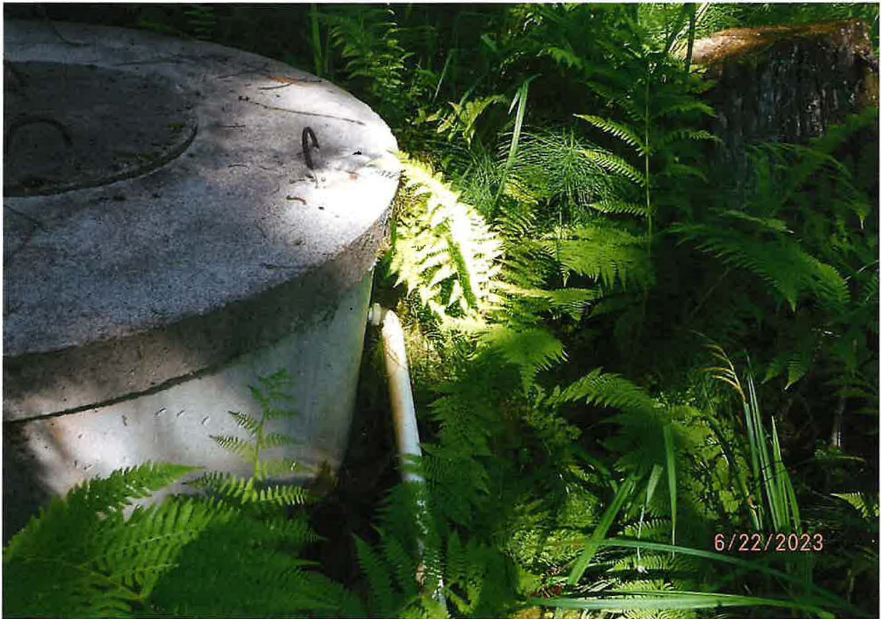
POD – 2 OF 2 SHALLOW HAND DUG GROUNDWATER WELLS (12 FT DEEP) WITH CONCRETE RINGS OVERFLOW PIPE FROM 14 FT HAND DUG WELL – MAIN LINE IS A BURIED GRAVITY FLOW PIPELINE
