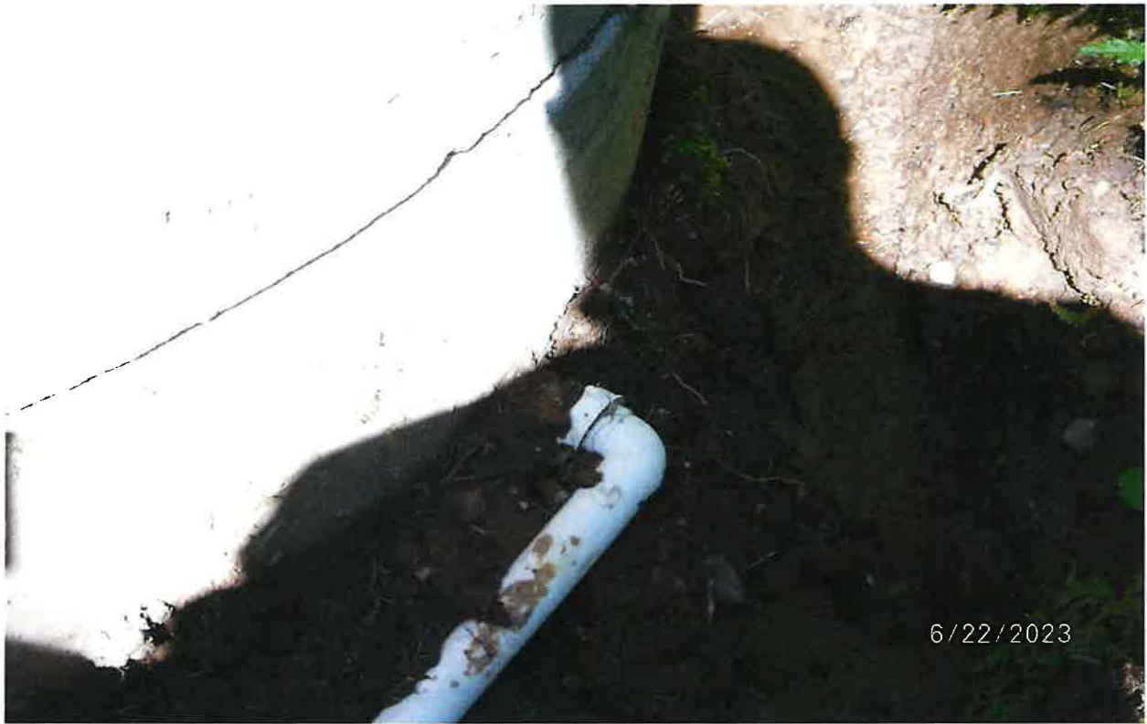
OVERFLOW PIPE FROM 14 FT HAND DUG WELL – MAIN LINE IS A BURIED GRAVITY FLOW PIPELINE
