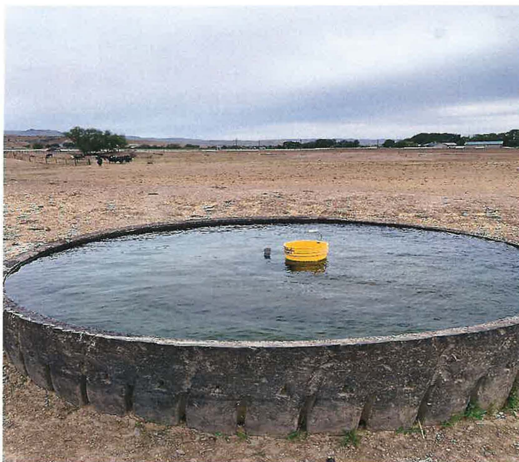
Fig. 10 - Stockwater trough South of the corral that is fed by the well in fig. 8.
