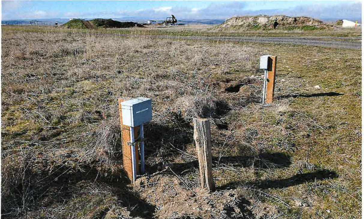
VACANT LOT 8, BLK 1 STUB IN & LOT 9 BLK 1 WITH HOME CHUKAR RUN SUBDIVISION PICTURE DEPICTS VACANT LOTS #8 BEFORE DRIVEWAY & #11 IN THE BACKGROUND
