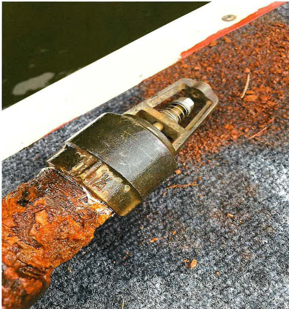
INTAKE PIPE WITH ¼ INCH SCREENED FOOT VALVE
