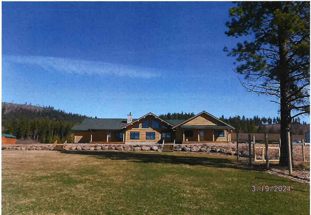
RESIDENCE LOCATED IN BETWEEN GREENHOUSE AND LODGE. THIS RESIDENCE IS ON THE 2 ND (SEPARATE) GROUNDWATER WELL (D0059576) SYSTEM COVERED BY DECREE WR 95-17566. PUMP CONTROL AND PRESSURE TANK LOCATED IN SAME PUMP STATION AS WR 95-17621, BUT ON A SEPARATE DISTRIBUTION SYSTEM.
