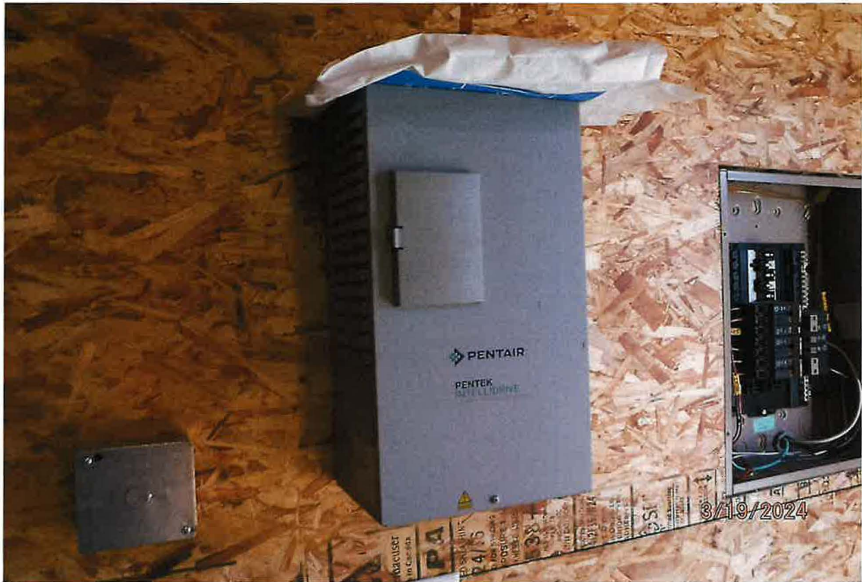
1 HP VFD PENTEK PUMP MOTOR INSTALLED ON WELL PUMP
