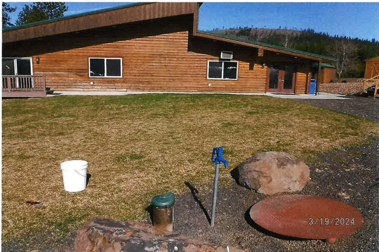
POD – LOCATED IN FRONT OF FACILITY ASSOCIATED WITH DOMESTIC POU
