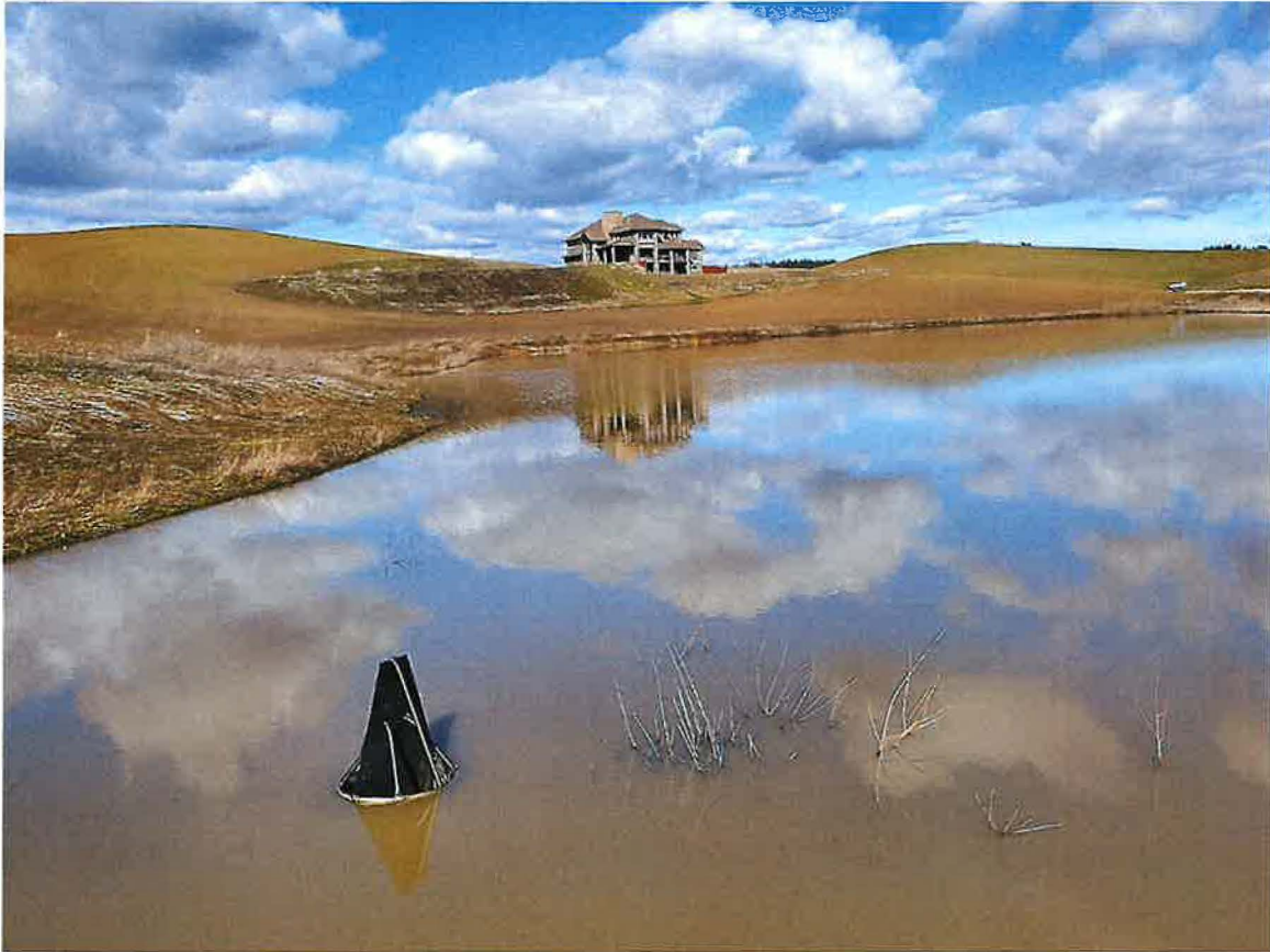
Overflow pipe at southwest corner of pond near outflow channel
