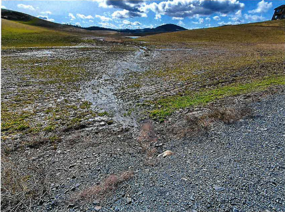
Culvert with natural flow of water from driveway
