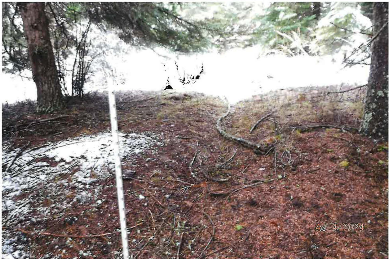
FIRE PROTECTION FROM STORAGE – BURIED 2 INCH POLY PIPELINE ROUTED 1,000 FT FROM POND TO VALVE; SLIGHT DEPRESSION IN PHOTO SHOWS EXCAVATION TRENCH LINE WITH SETTLED SOILS
