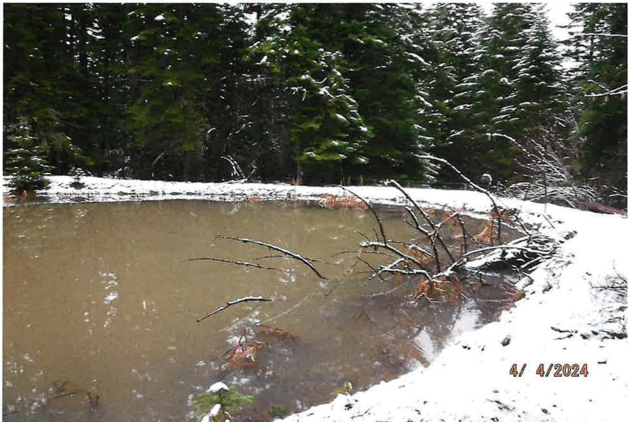
POU – STORAGE POND WITH EARTHEN DAM; NO OVERFLOW DEVICES CONSTRUCTED FOR SMALL POND
