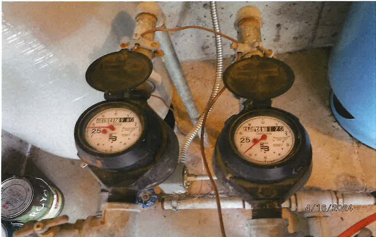
RECORDALL MODEL 25 FLANGED VELOCITY STYLE FLOW METERS – USED TO CAPTURE INSTANTANEOUS FLOW DURING BENEFICIAL USE FIELD EXAM.
