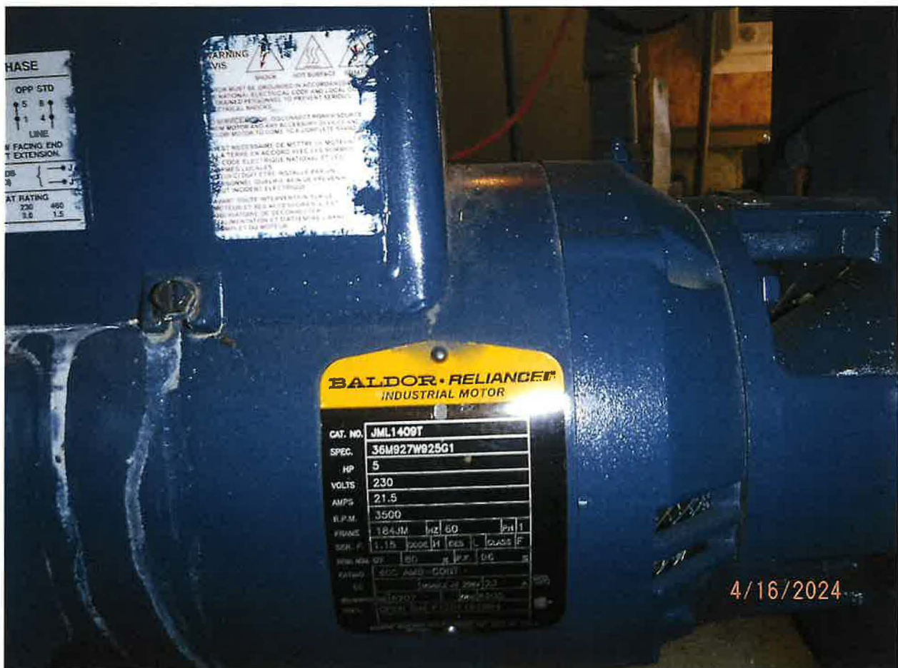
STA-RITE PUMP WITH 5 HP BALDOR-RELIANCE CENTRIFUGAL PUMP USED TO SERVE COMMUNITY SYSTEM FROM THE STORAGE RESERVOIR
