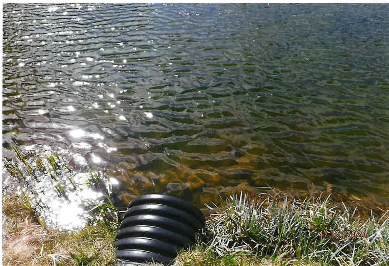
18 INCH CORRUGATED PIPE ALLOWS WATER FROM UPPER POND TO FLOW INTO LOWER POND
