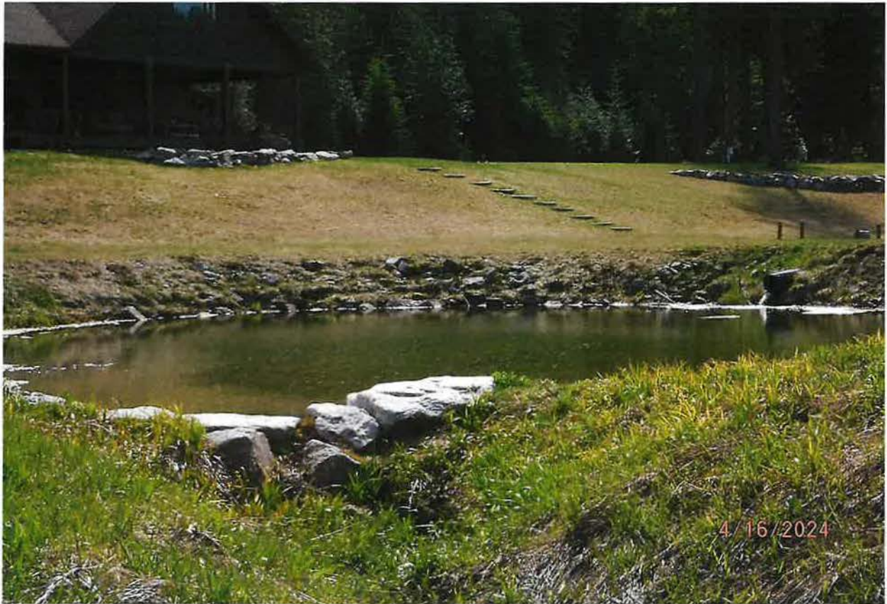
ROCKED OVERFLOW CHANNEL FROM LOWER POND ROUTES TO NEARBY STREAM
