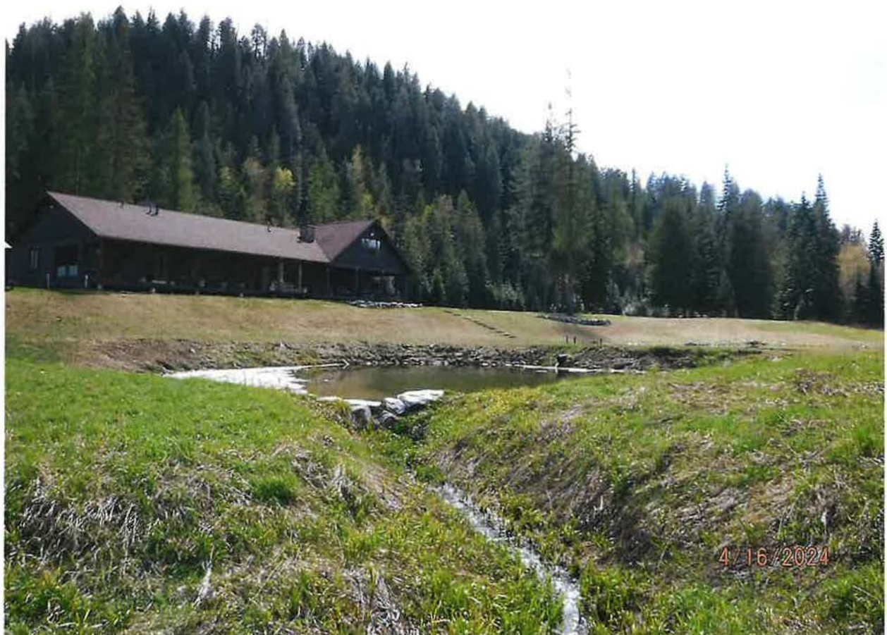
ROCKED OVERFLOW CHANNEL FROM LOWER POND ROUTES TO NEARBY STREAM
