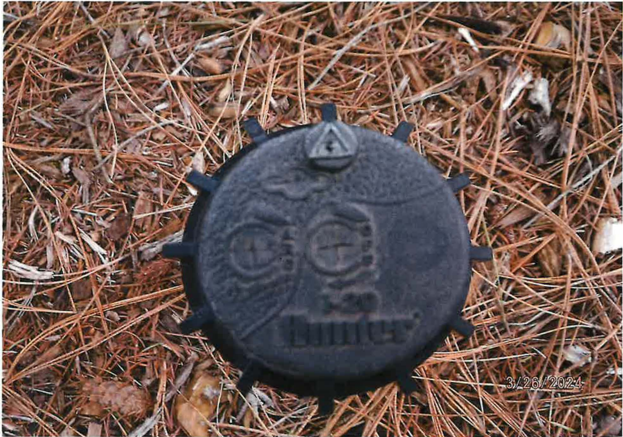
IRRIGATION POU – EXAMPLE OF PRESSURIZED SPRINKLER USED FOR ZONE IRRIGATION – HUNTER I-20 MODEL
