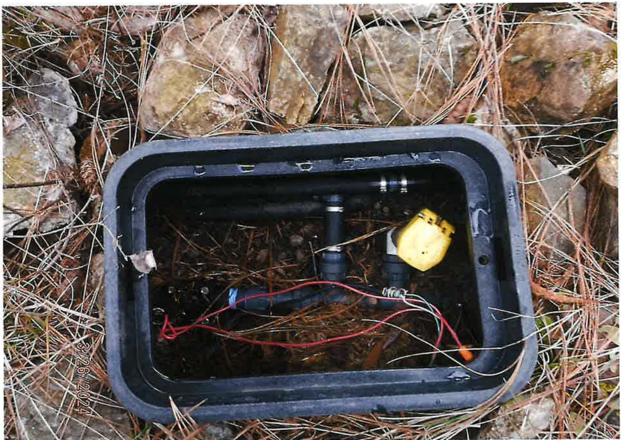
IRRIGATION POU – EXAMPLE ZONE CONTROL BOX
