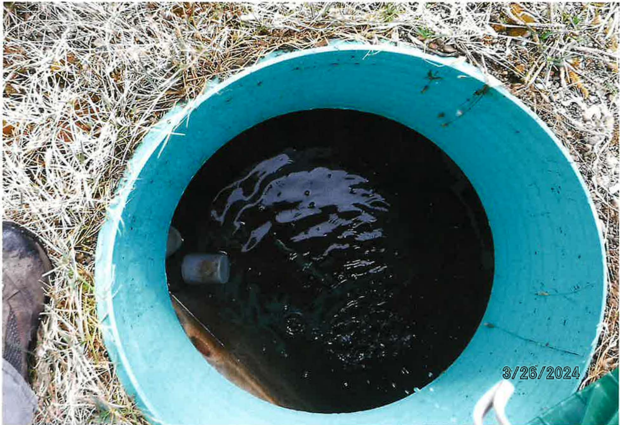
1,700 GAL STORAGE CISTERN WITH 1.5 HP PENTEK TRANSFER PUMP USED FOR PRESURIZED IRRIGATION SYSTEM: 9 ZONES WITH 6 HEADS PER ZONE
