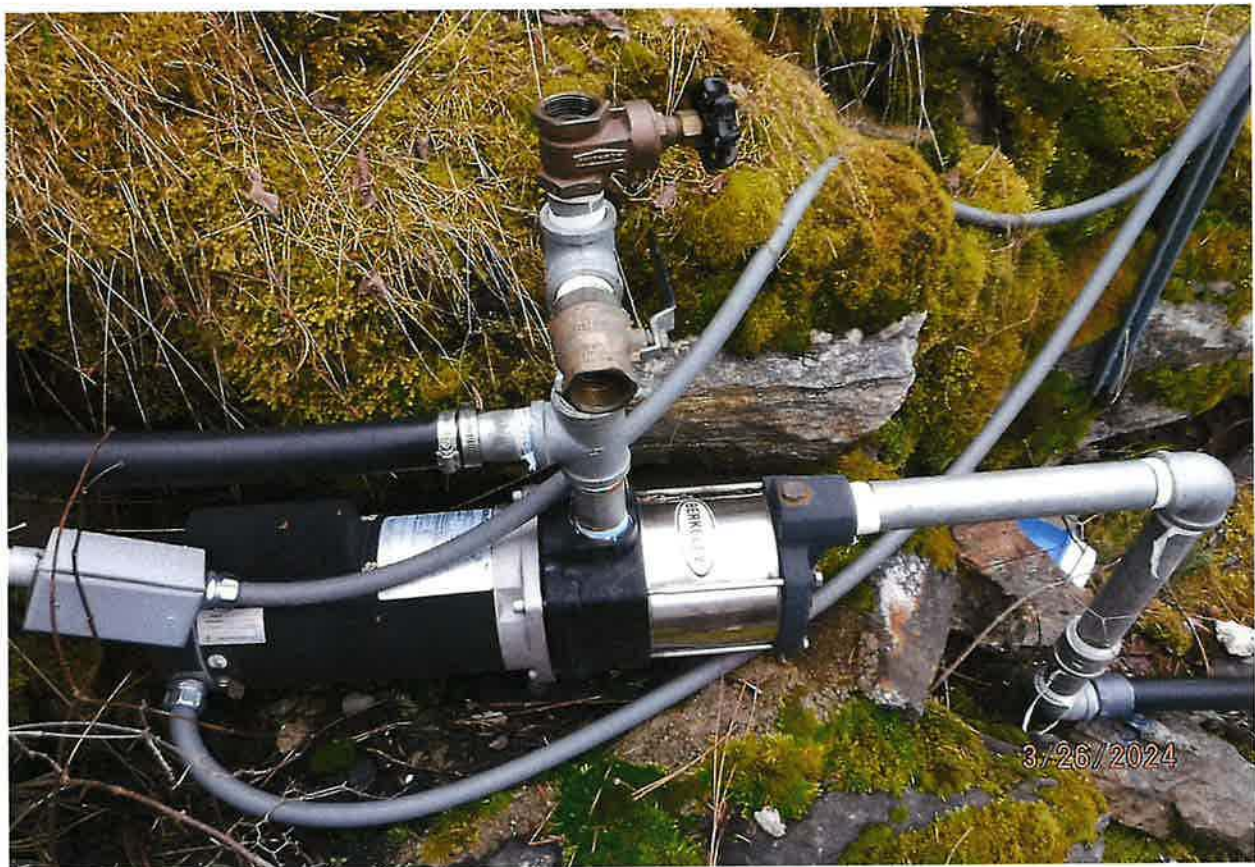
POD – 2 HP SINGLE PHASE BERKELEY PUMP MODEL B82456-01 / MOTOR # 196553
