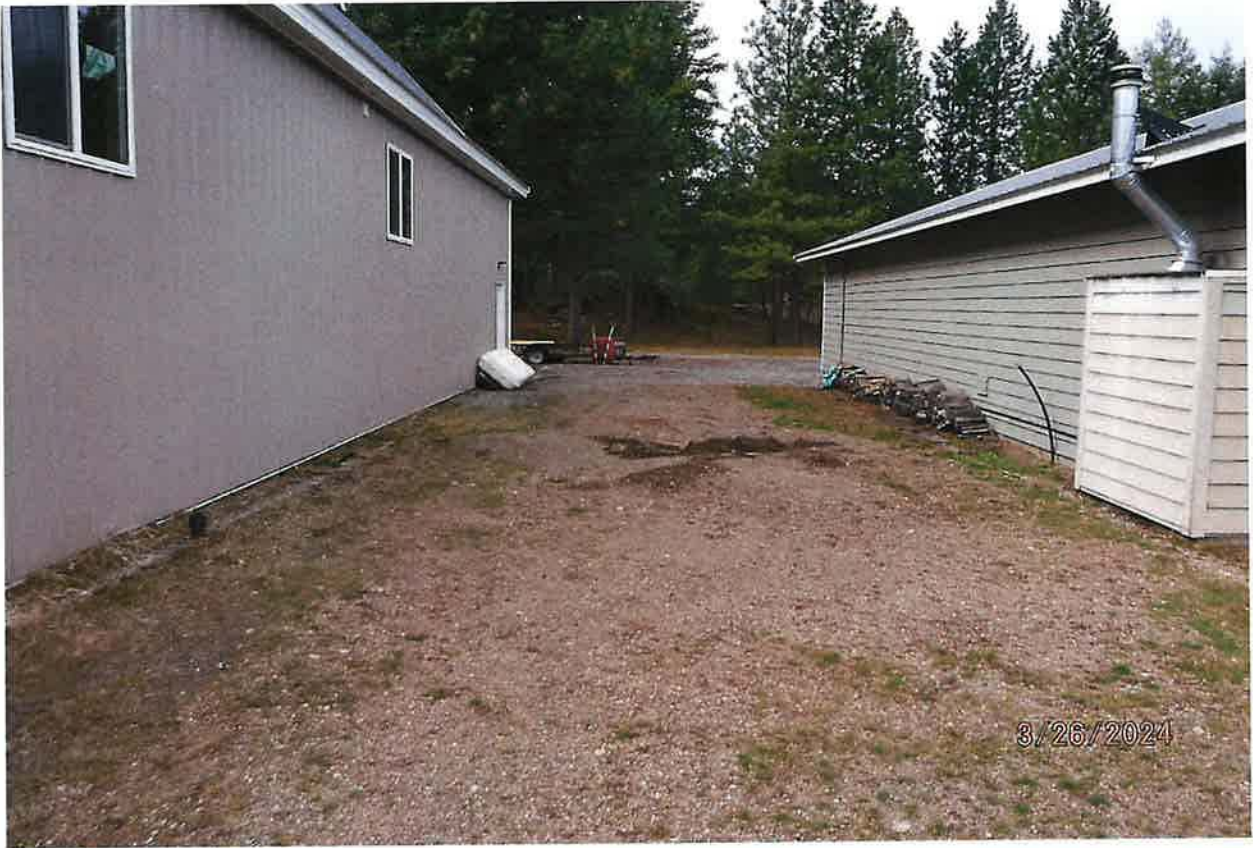
AREA BETWEEN GARAGE AND BARN IS NOT IRRIGATED
