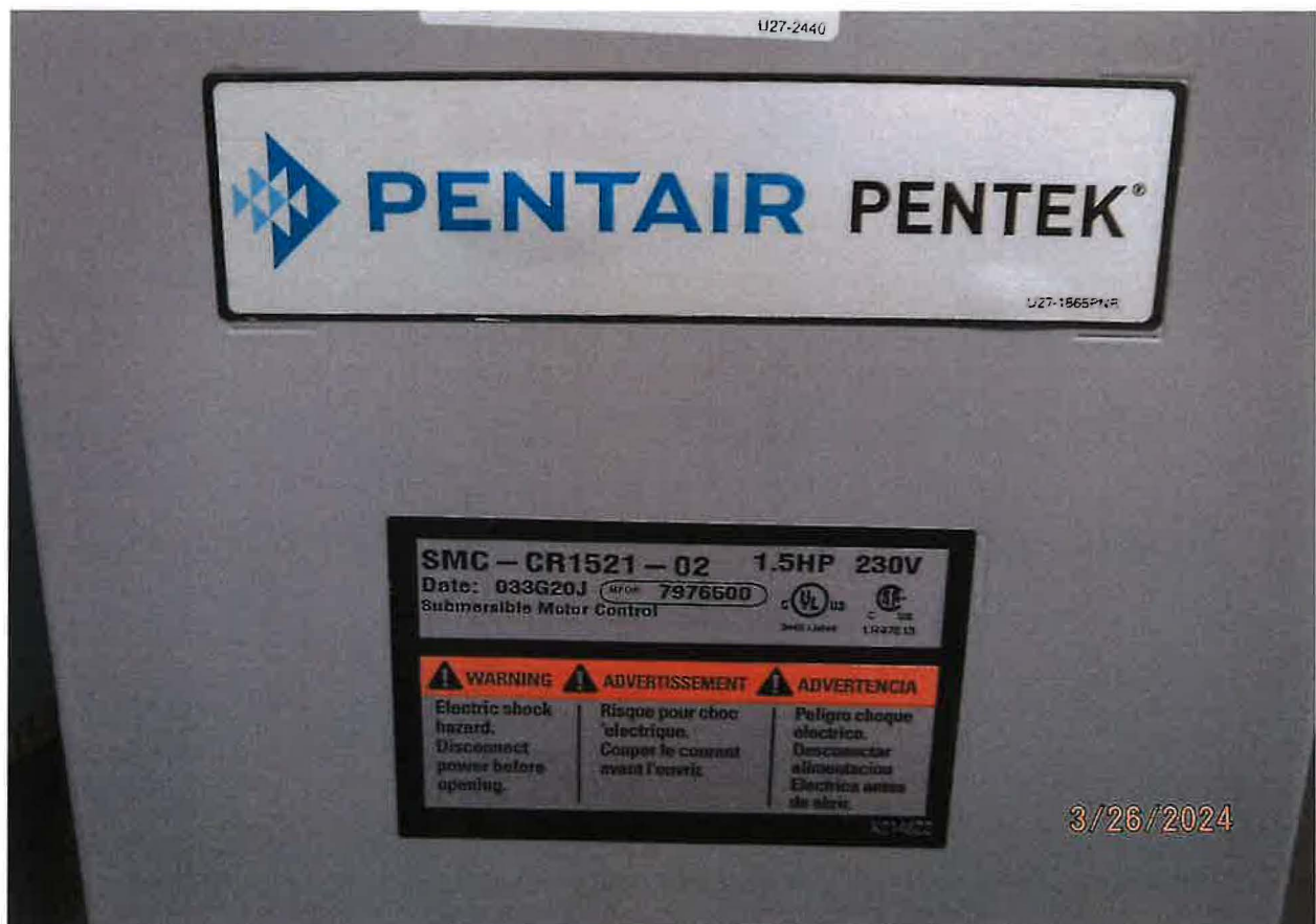
1,700 GAL STORAGE CISTERN WITH 1.5 HP PENTEK TRANSFER PUMP USED FOR PRESURIZED IRRIGATION SYSTEM: 9 ZONES WITH 6 HEADS PER ZONE
