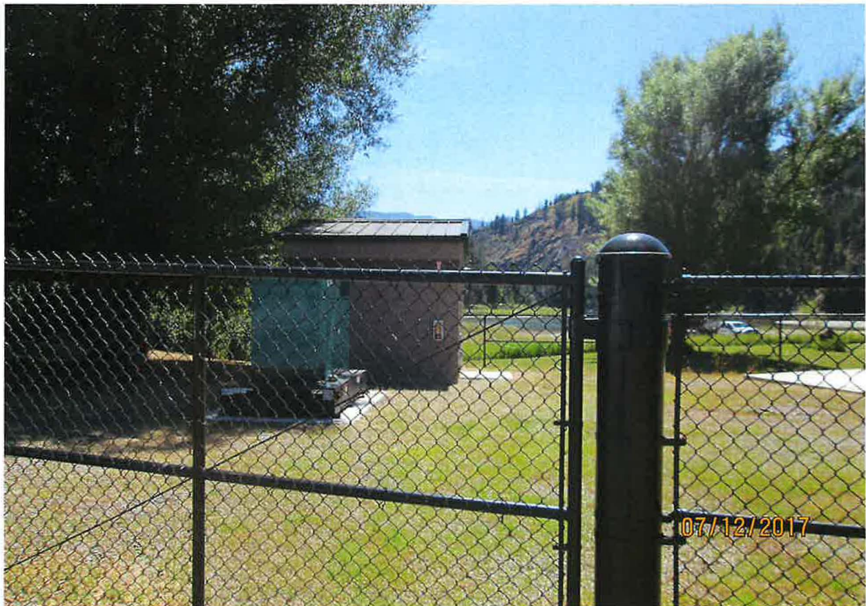
KOOTENAI RIVER CONVEYANCE SYSTEM PUMP STATION
