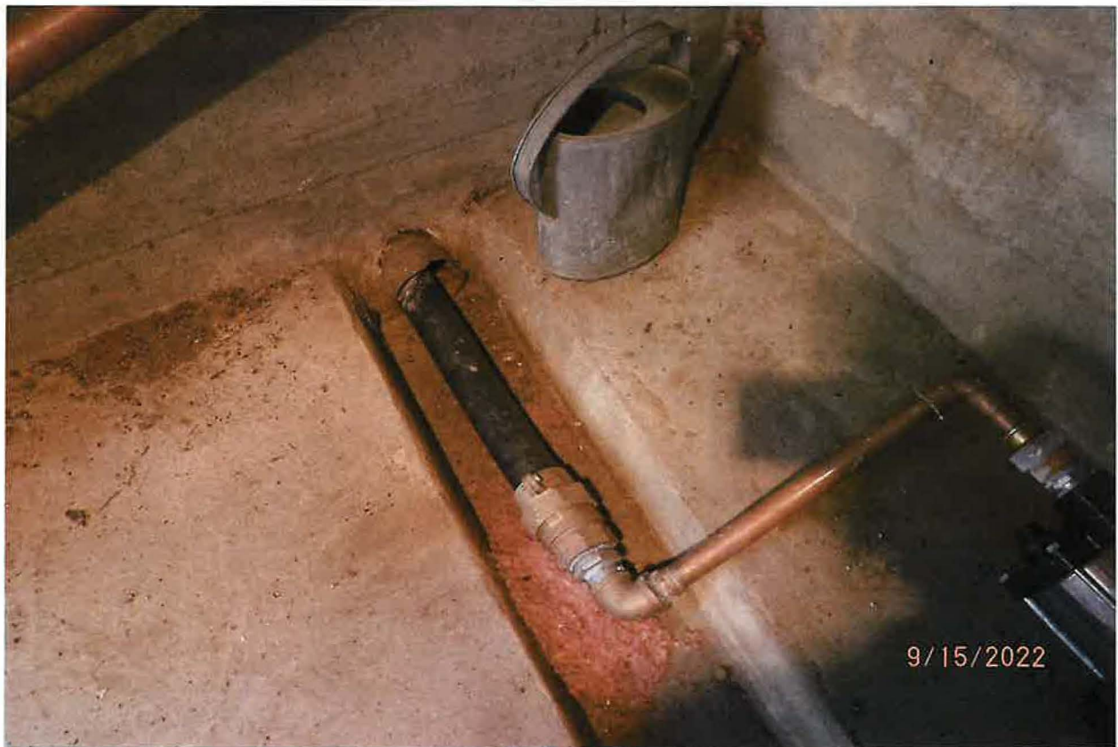
INFLOW PIPE FROM LAKE
