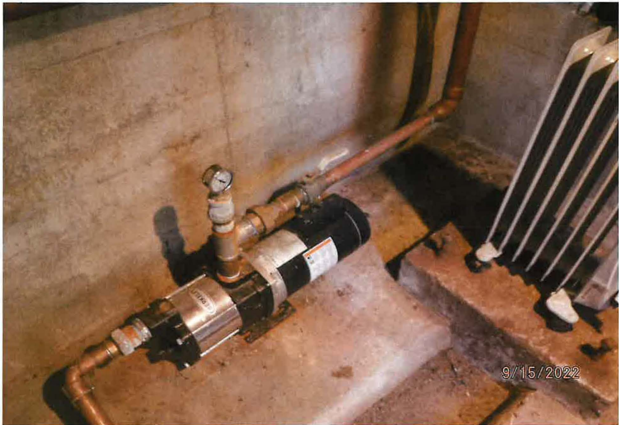
2 HP PUMP MOTOR, SINGLE PHASE 3,450 RPM BERKELEY PUMP WITH PENTEK MOTOR
