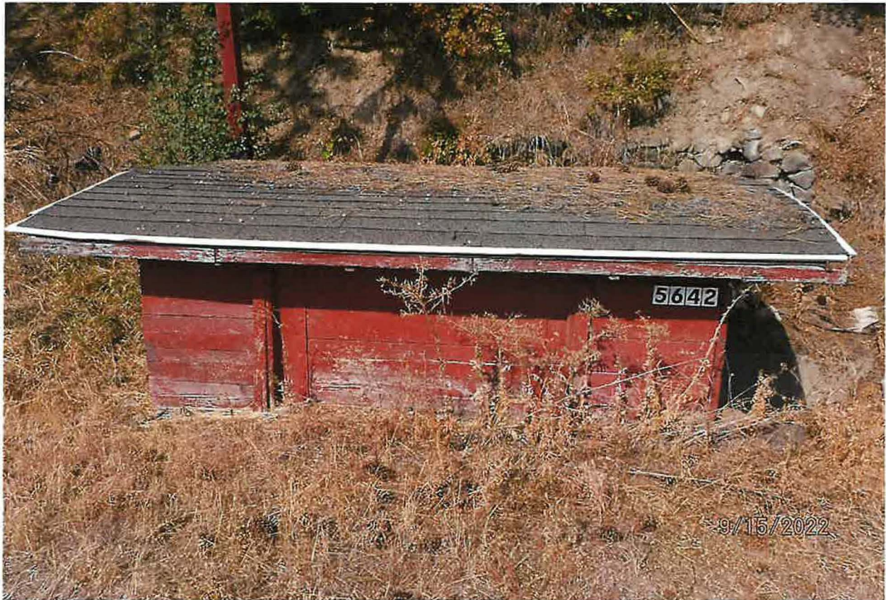
POD – PUMPHOUSE – SURFACE WATER SYSTEM FIRST DAYLIGHTS IN THIS PUMP STATION
