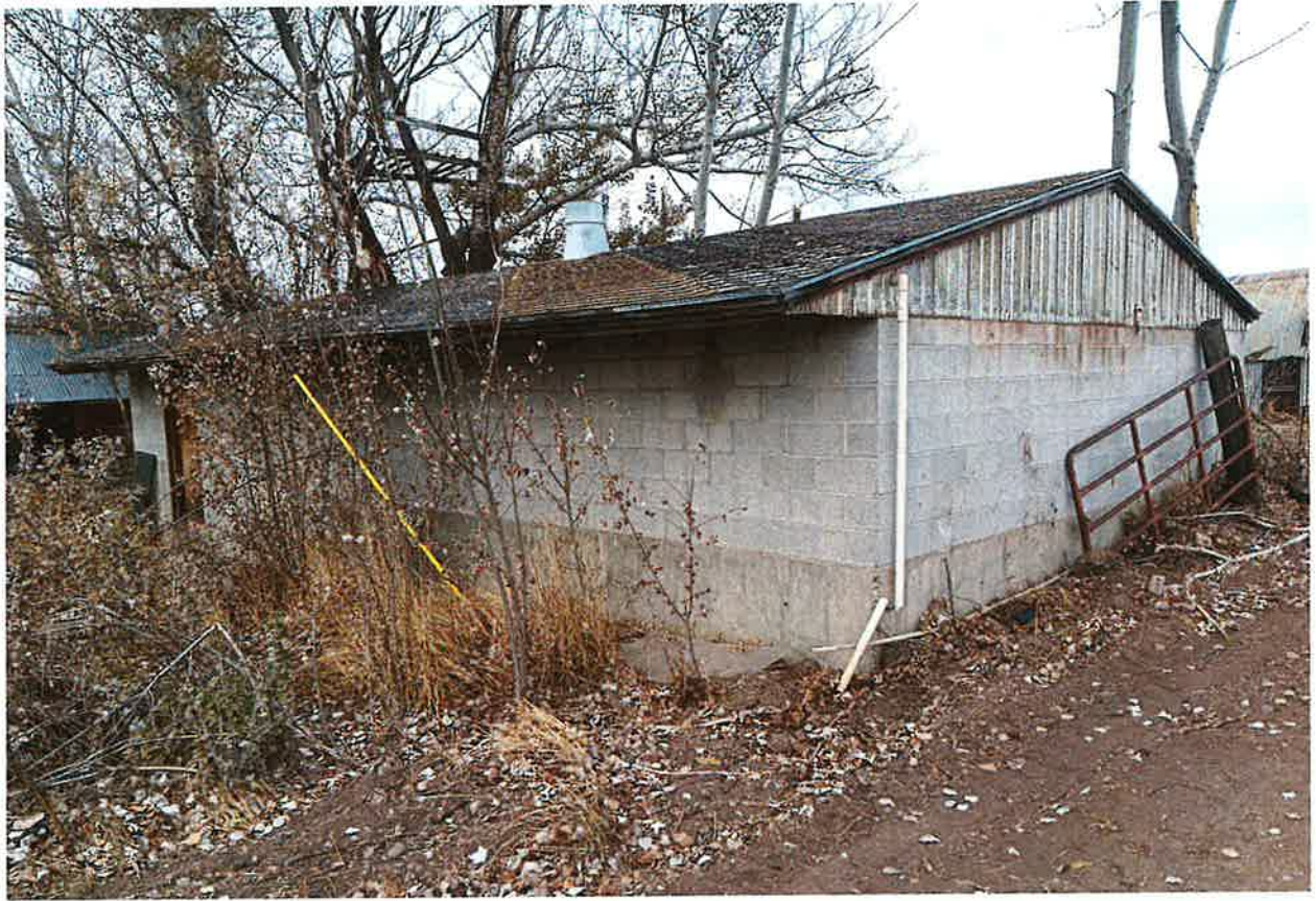
Main Pump House (Taken 11/22/24)
