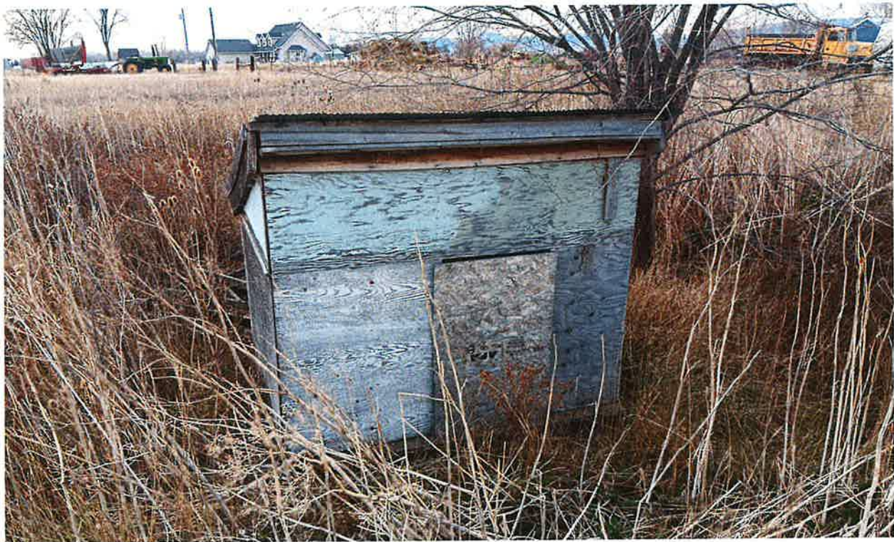
Low Water Pump House (Taken 11/22/24)
