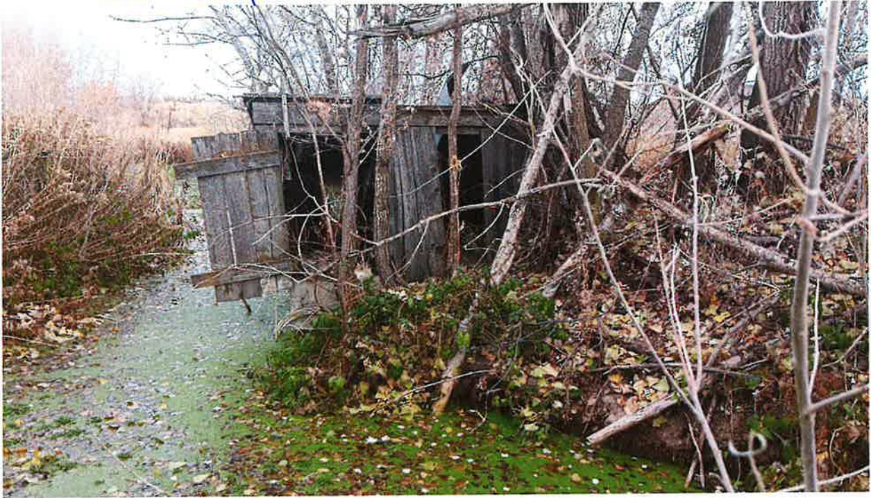
Old Pump House (Taken 11/22/24)
