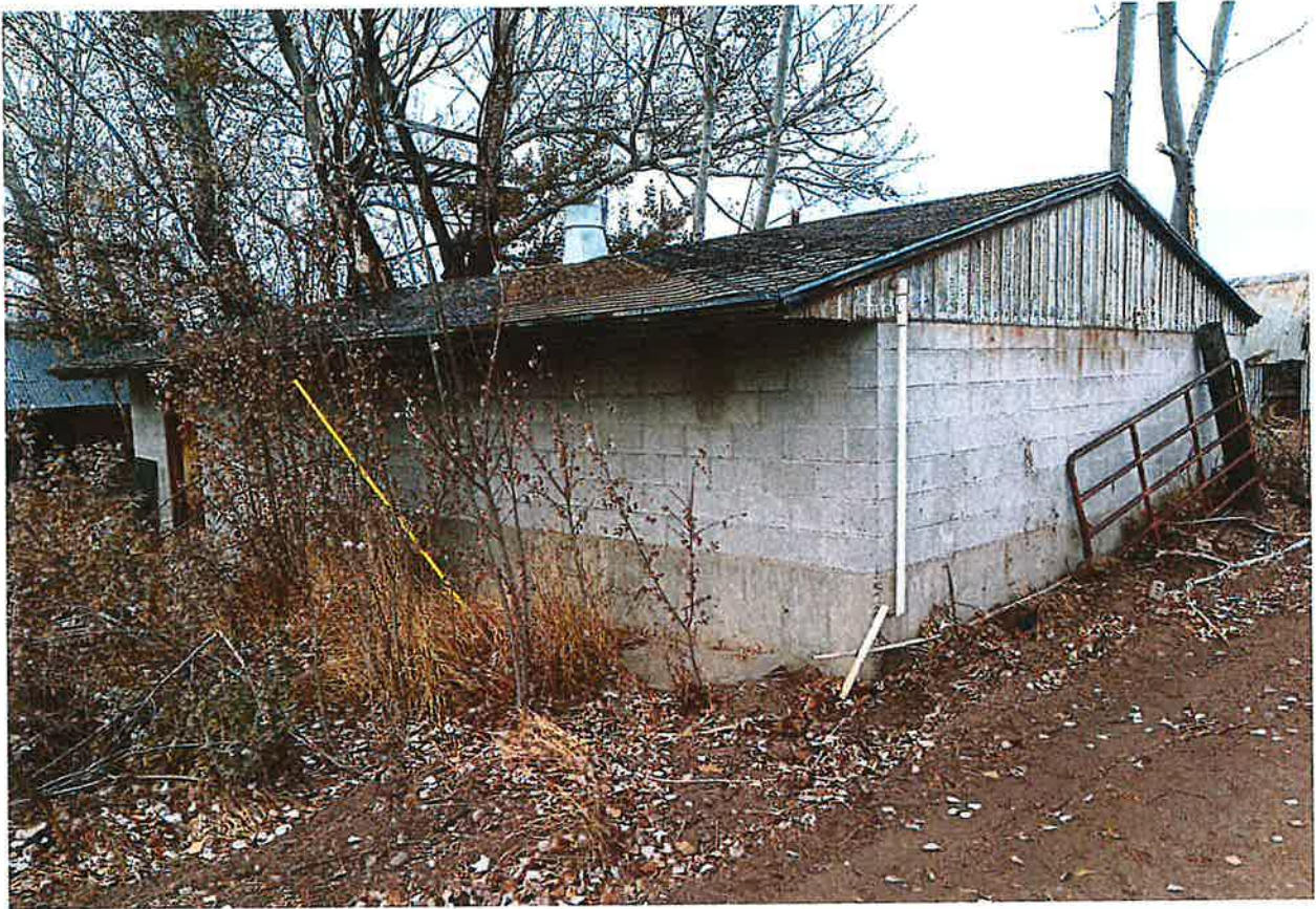
Main Pump House (Taken 11/22/24)
