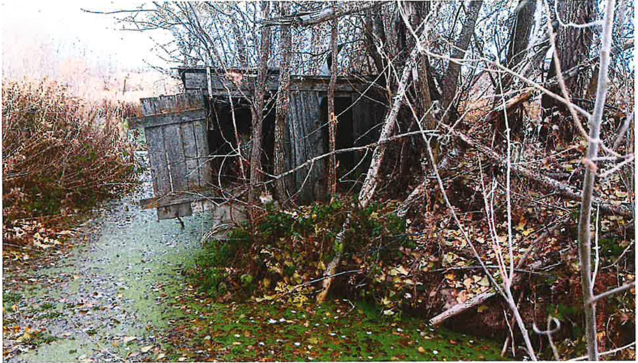
Old Pump House (Taken 11/22/24)
