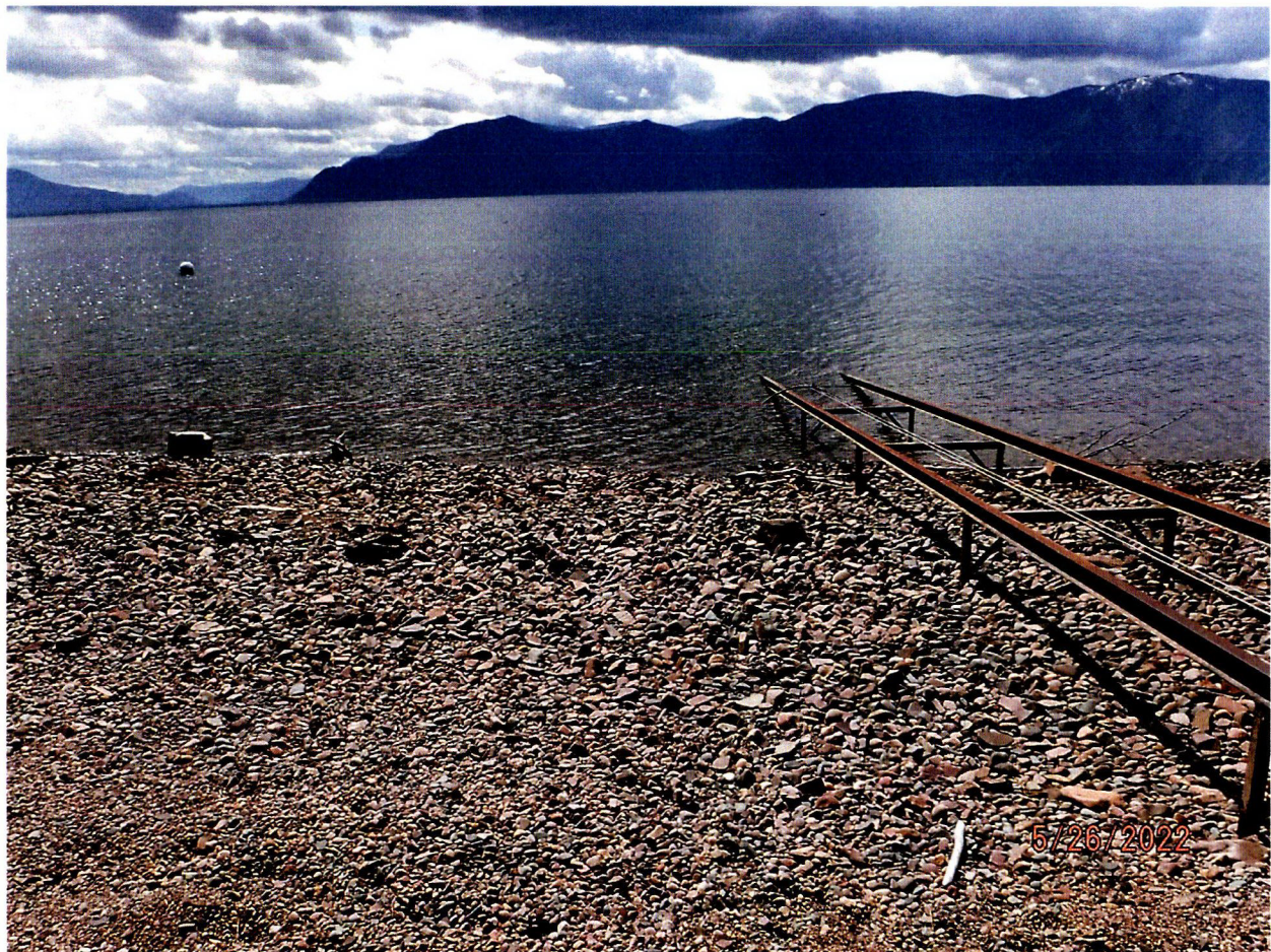
POD – BURIED POLY PIPE TO PUMP IN LAKE ROUTED ALONG SIDE BOAT LAUNCH
