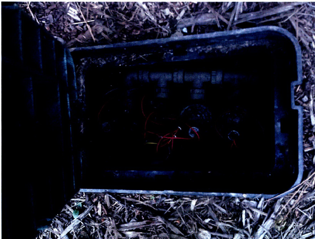
Photos 3 & 4- Control boxes 1 & 2, each with 4 control valves (zones).
