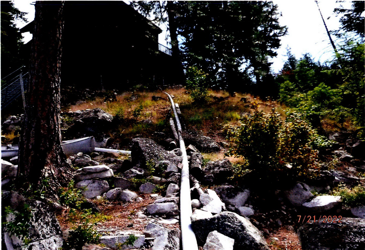
1 1/4 INCH POLY PIPE ROUTED INSIDE 4 INCH PVC PIPE FOR PROTECTION
