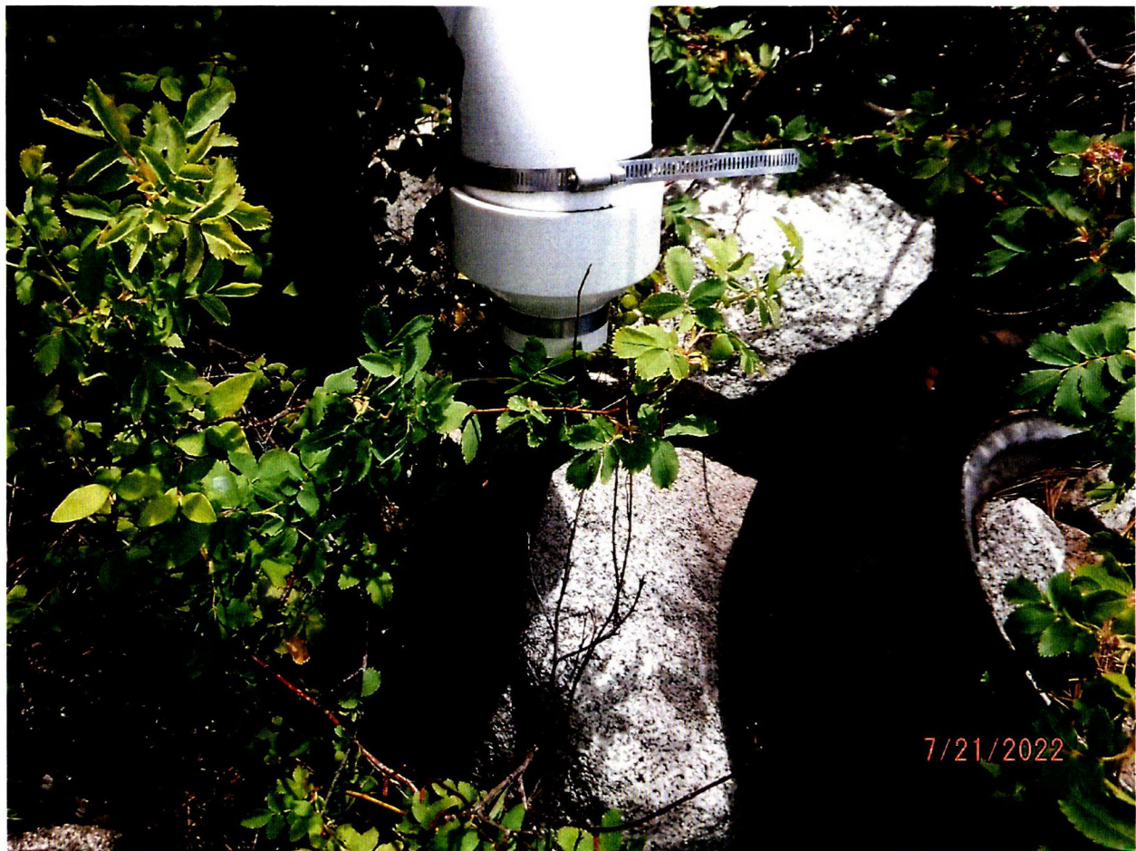
1 1/4 INCH POLY PIPE ROUTED FROM POD UP GRADE TO RESIDENCE
