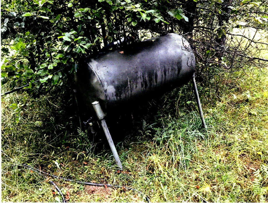
Photo 3- Water tank with 2" plastic line from pump attached to fill at the top.
