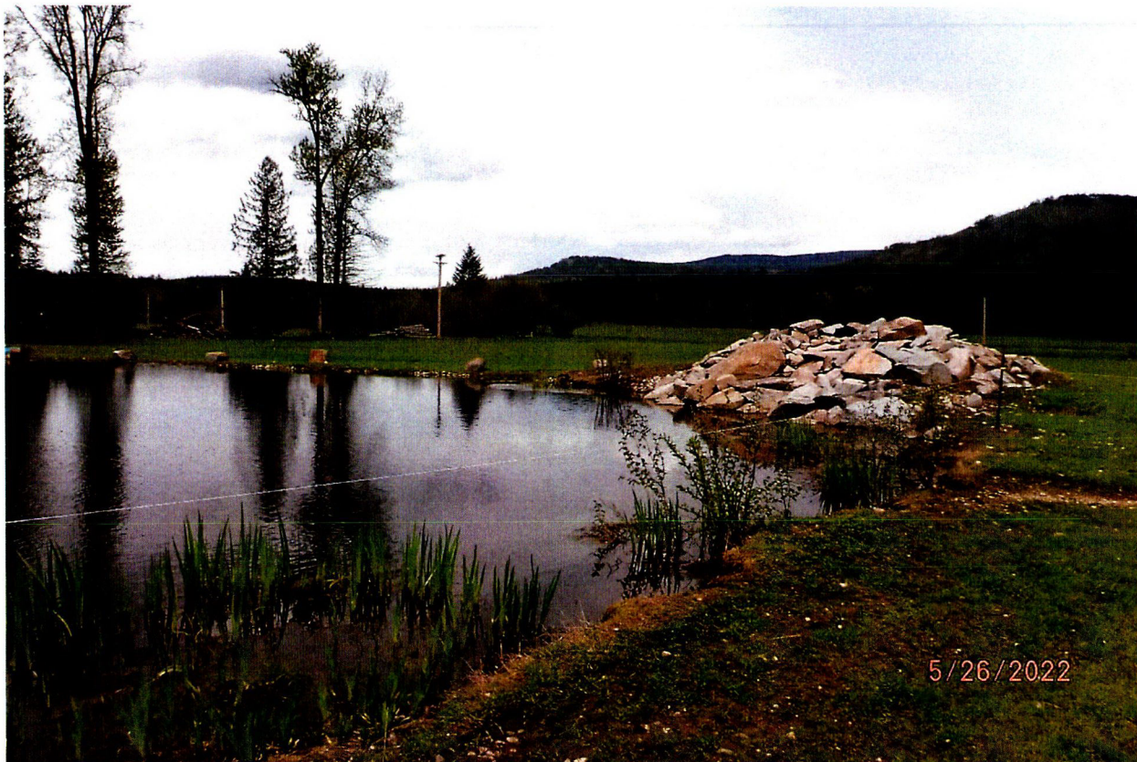
SEASONAL OVERFLOW DISCHARGES VIA MINOR OVERFLOW CHANNEL
