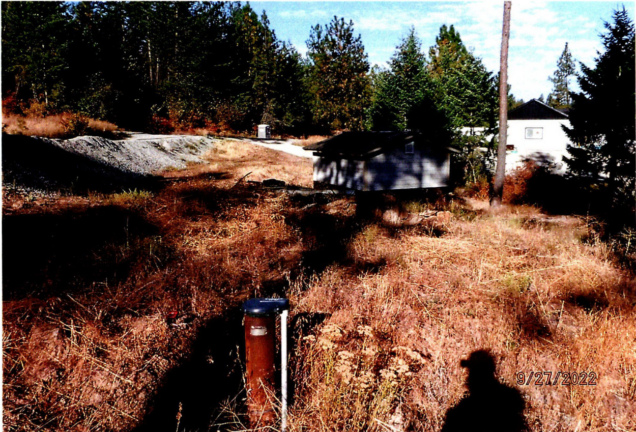
POD – GROUNDWATER WELL WITH PUMP HOUSE IN BACKGROUND
