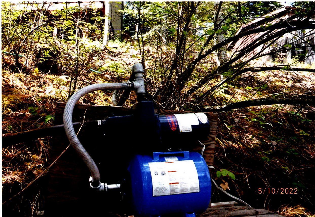
PENTEK ¾ HP PUMP INSTALLED IN DIVERTING WORKS
