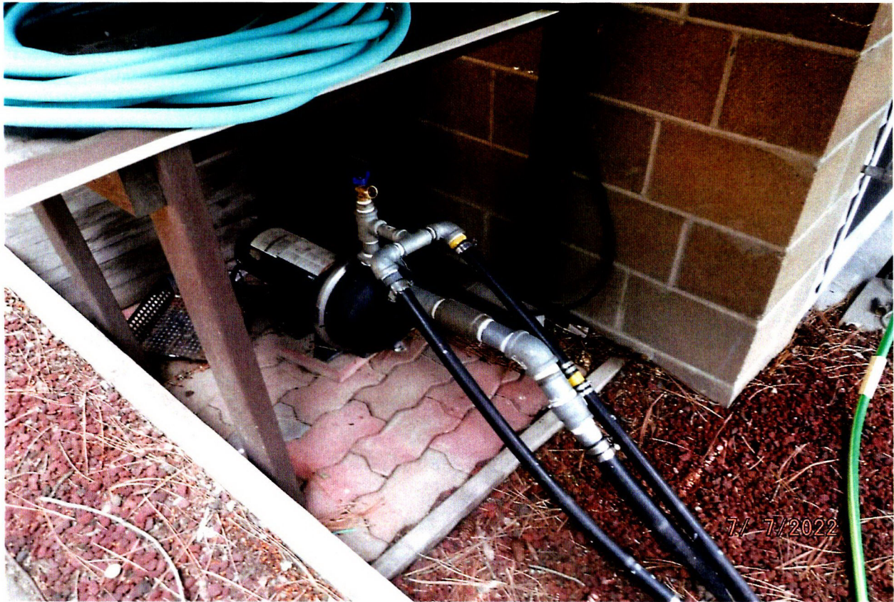
DIVERTING WORKS – CRAFTSMAN PUMP AND 2EA IRRIGATION ZONE SERVICE PIPES
