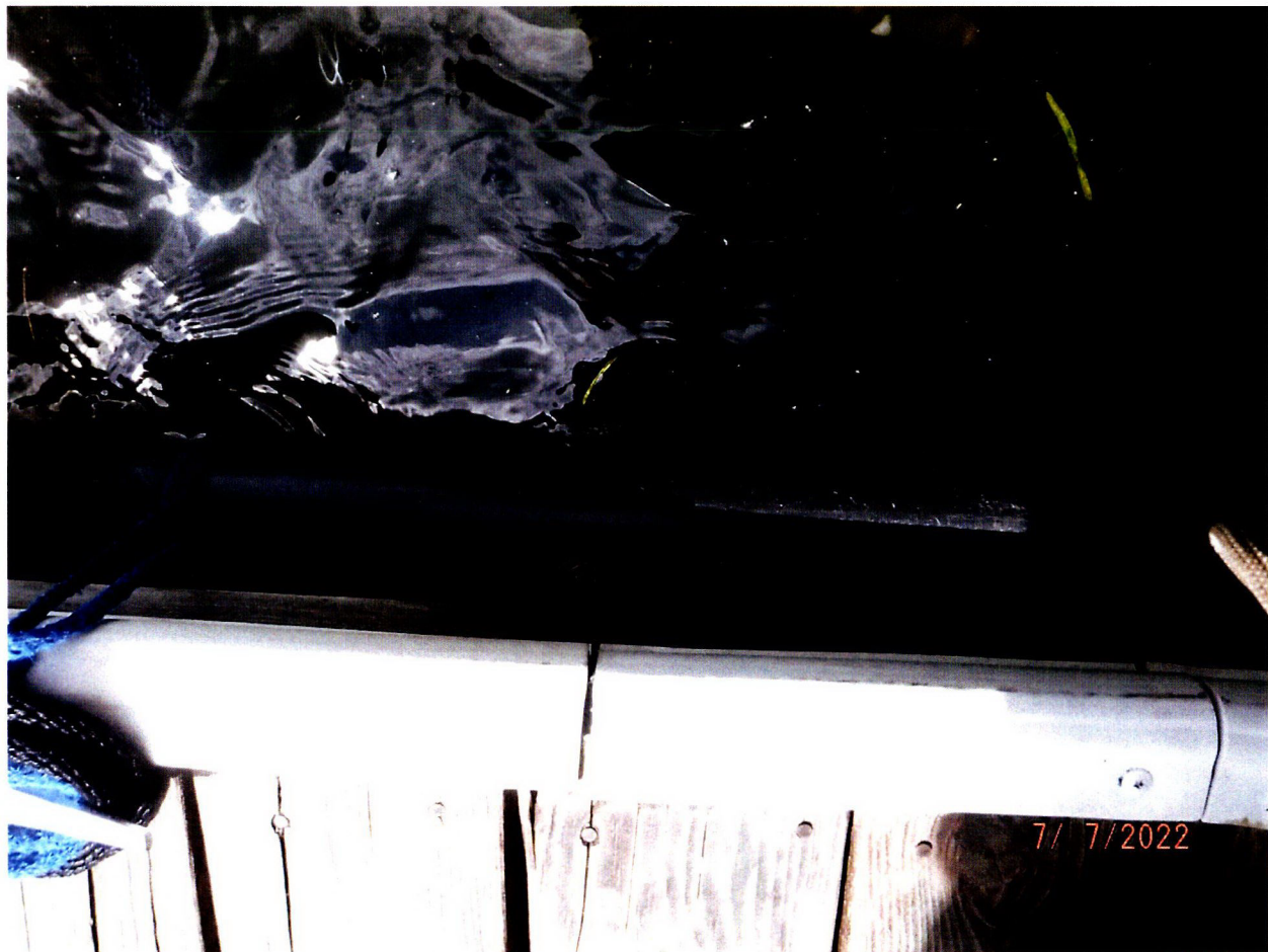
1 ½ INCH POLYPIPE INTAKE LINE SECURED TO LENGTH OF DOCK
