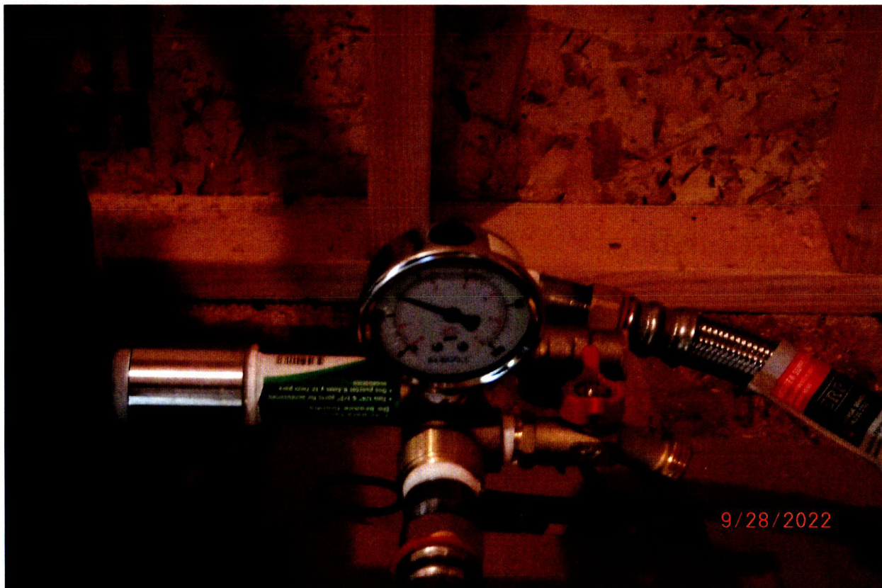
PRESSUER VALVE NOT REGISTERING FLOWING WATER – SYSTEM SHUT DOWN FOR SEASON
