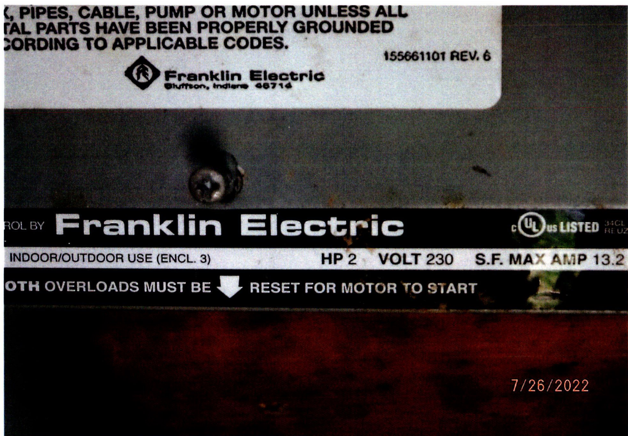
FRANKLIN ELECTRIC 2 HP PUMP MOTOR INSTALLED IN WELL
