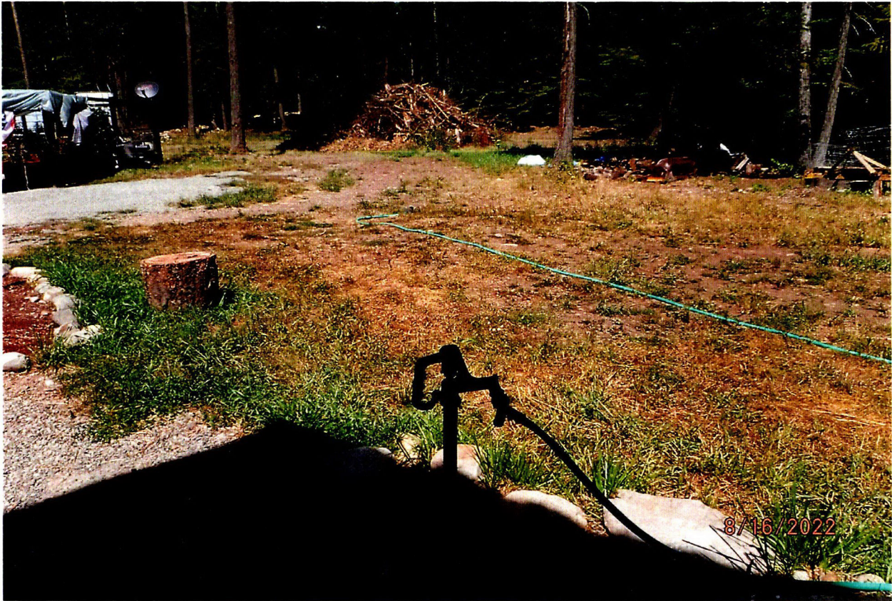
POU – FROST FREE HYDRANT & HOSE TO SPRINKLER FOR SMALL SCALE IRRIGATION UP TO ½ ACRE
