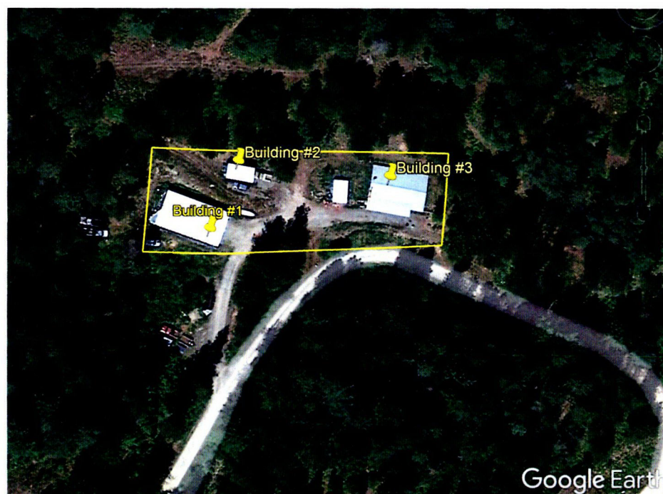
Figure 1.4- Buildings identification image sent to applicant.
