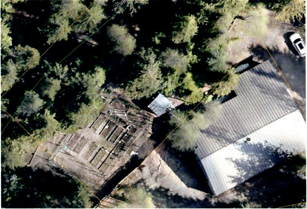
Figure 3- Bonner County map- aerial image of the southern portion of the permit holder's parcel (domestic POU) with garden beds visible.
