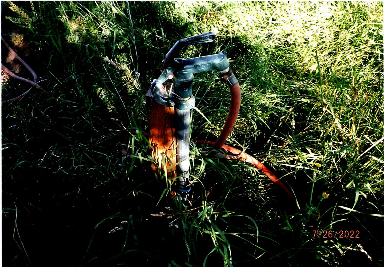
DOMESTIC USE IRRIGATION FROM 2EA FROST-FREE HYDRANTS
