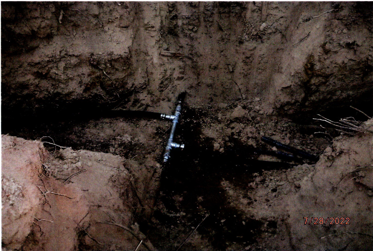
MAIN SERVICE LINE ROUTING THROUGH LT 16 FROM WELL TO LT 4, 2EA STUB-INS TEE OFF MAIN LINE
