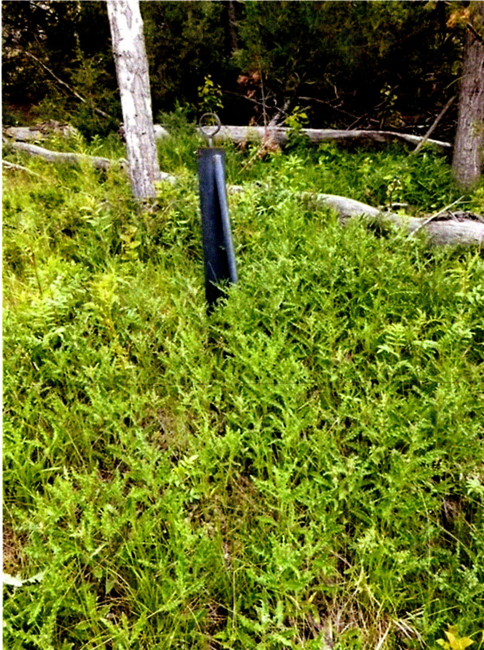
Vertical standpipe used to access outlet valve on cistern.
