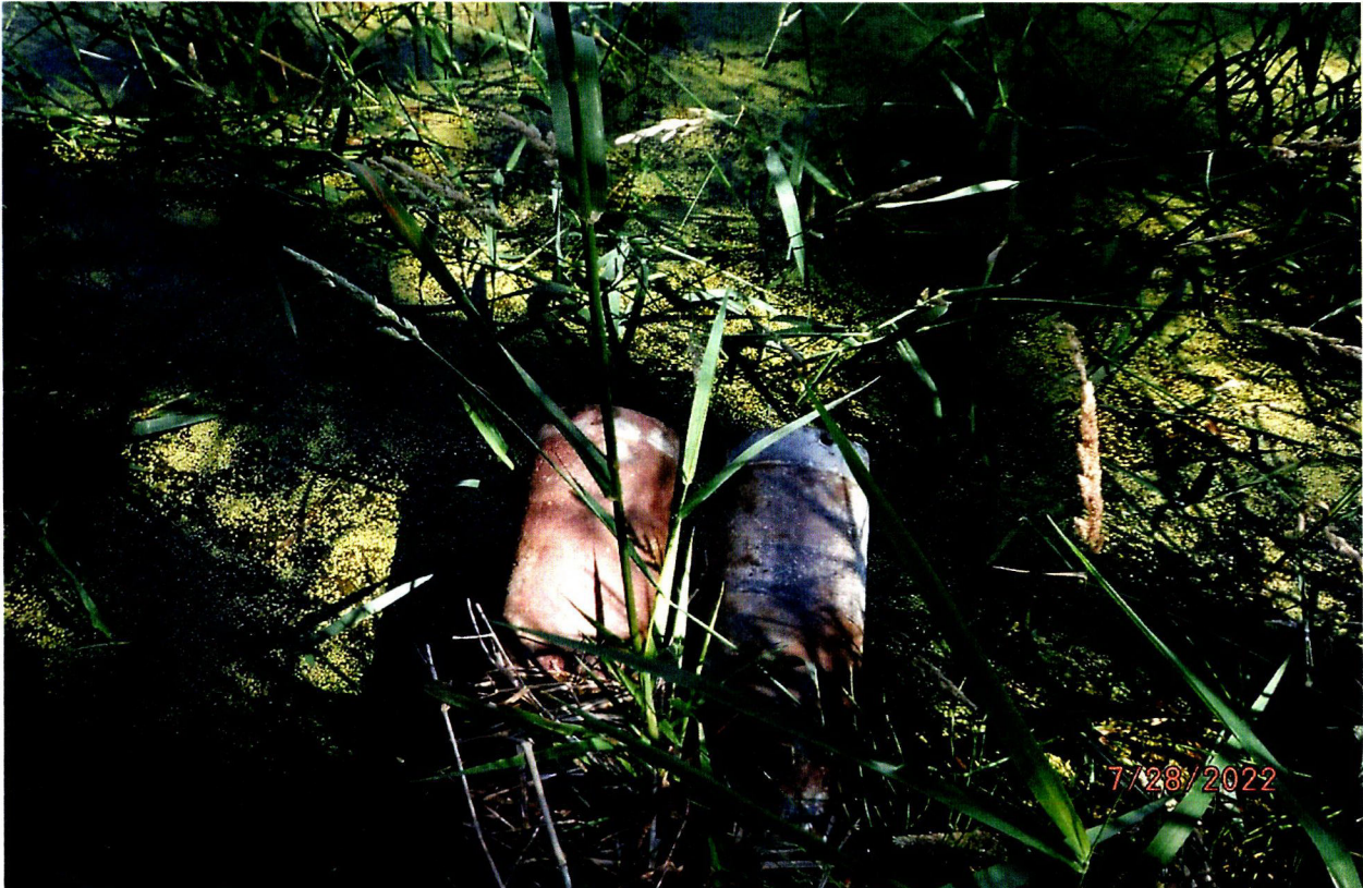
EARTHEN POND DAM WITH 2EA OVERFLOW PIPES INSTALLED
