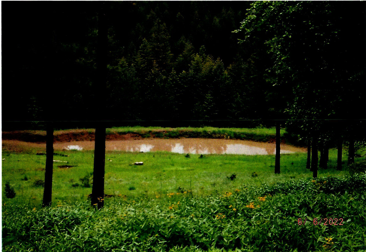
POD – EARTHEN POND DAM IMPOUNDS SURFACE RUNOFF WATER
