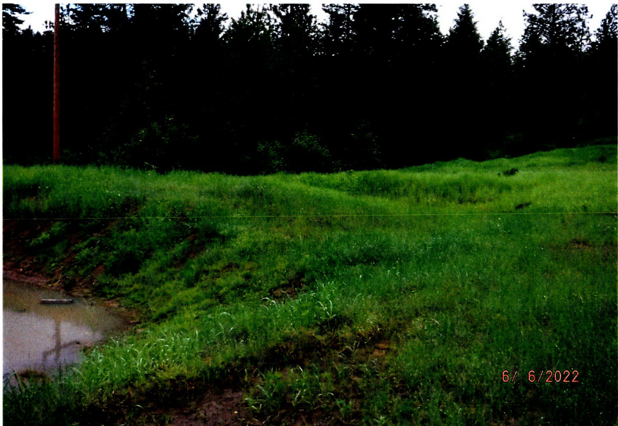
EARTHEN OVERFLOW DISCHARGE CHANNEL
