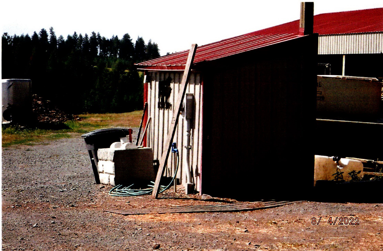
PUMP STATION HOUSES PRESSURE TANK FOR STOCKWATER SYSTEM
