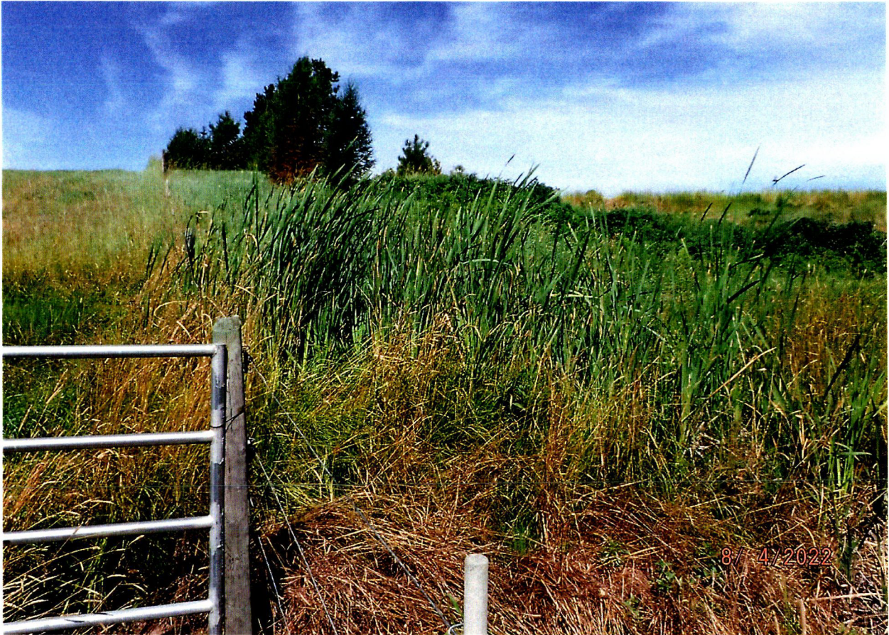
DRAIN TILE INSTALLED FROM SPRING FIELD TO CISTERN
