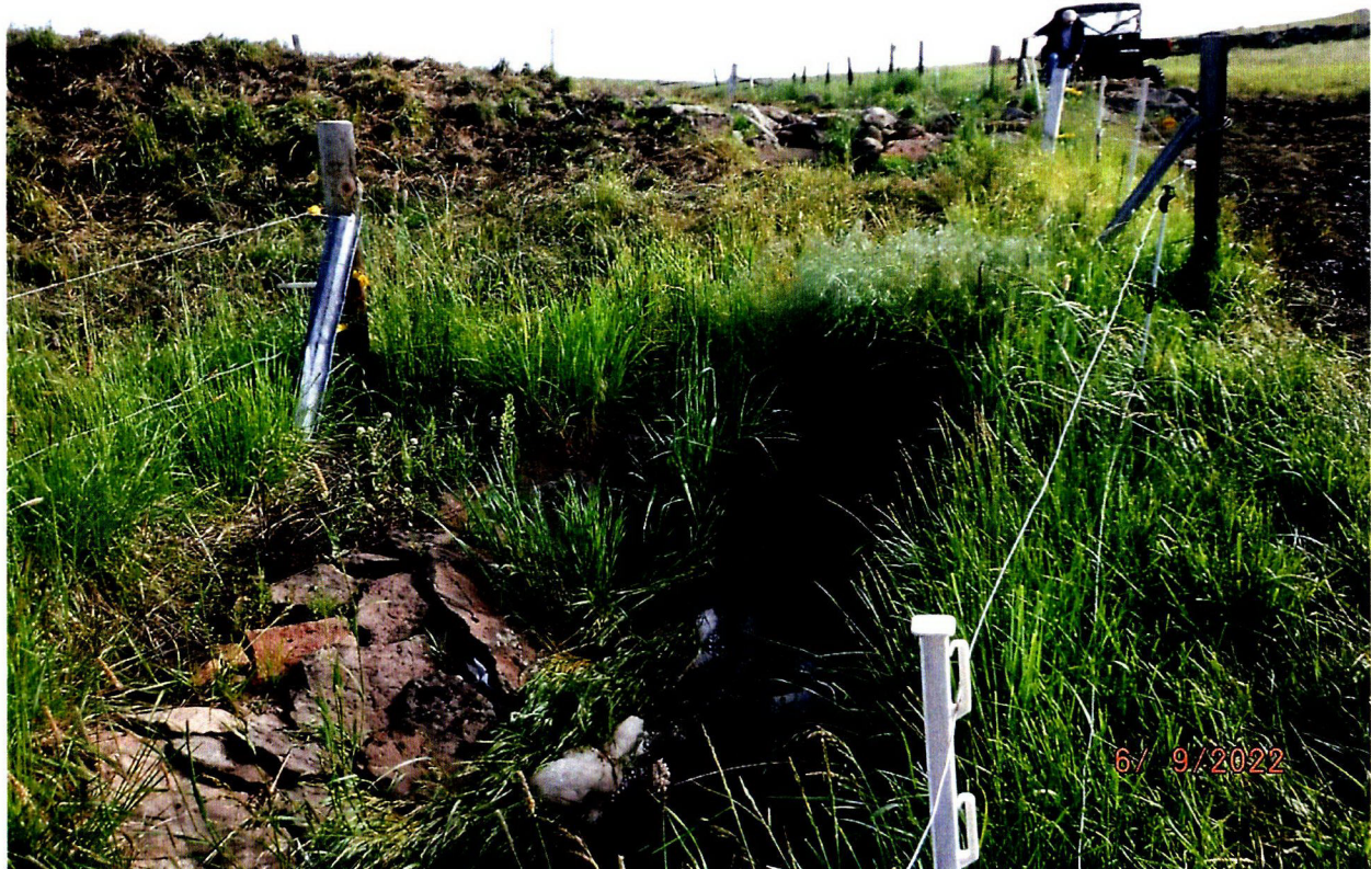
ROCKED OVERFLOW CHANNEL AND PIPE ROUTES DISCHARGED WATER BACK TO STREAM CHANNEL
