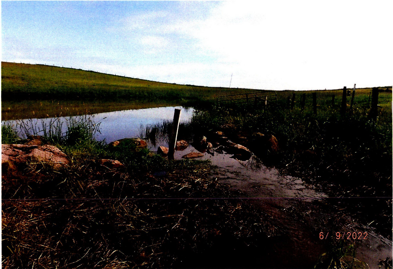
ROCKED OVERFLOW CHANNEL ON SE CORNER OF POND
